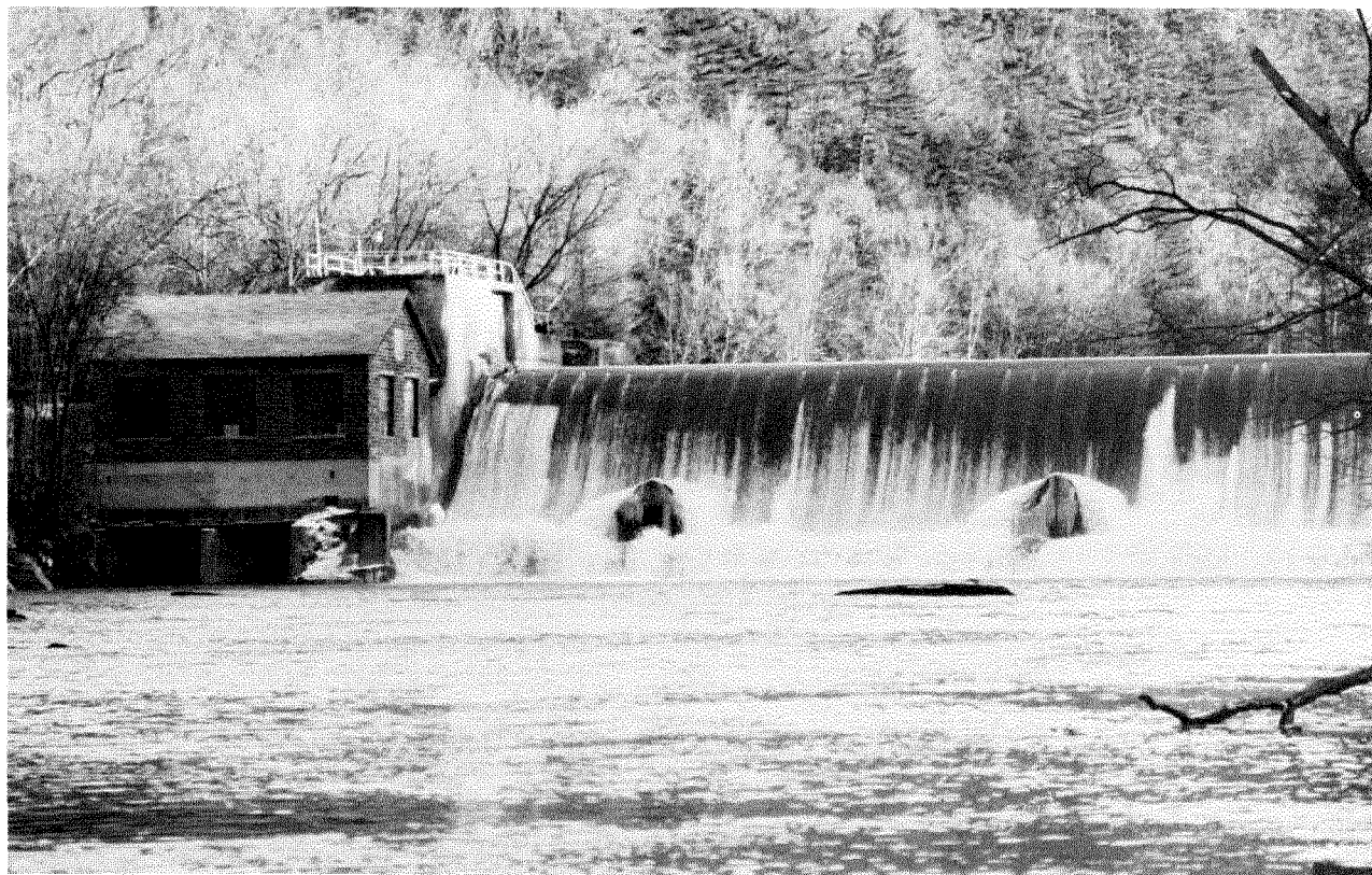
Springville Dam on Cattaraugus Creek
