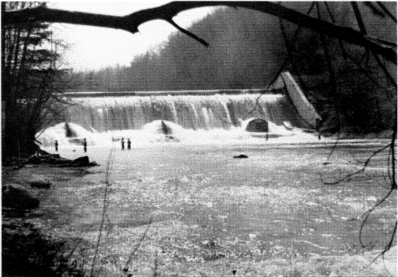
Springville Dam on Cattaraugus Creek
