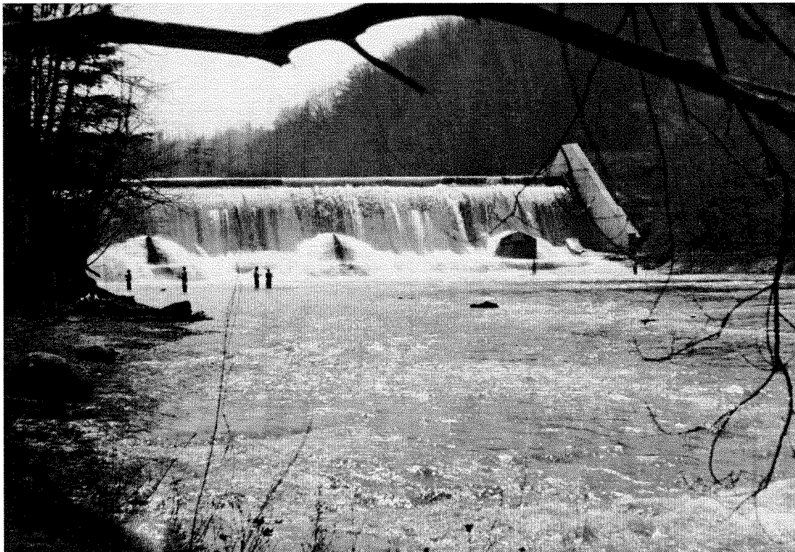
Springville Dam on Cattaraugus Creek
