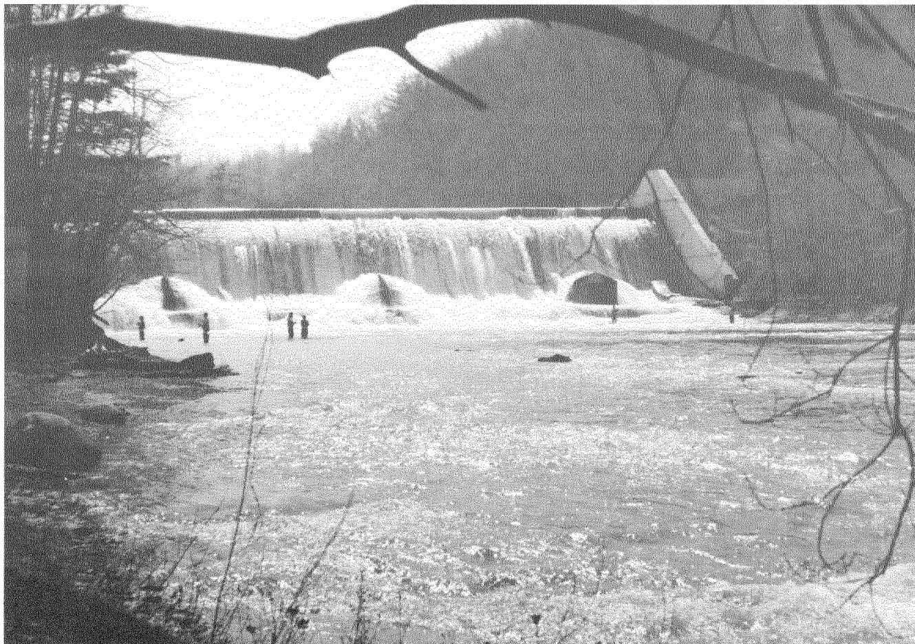
Springville Dam on Cattaraugus Creek
