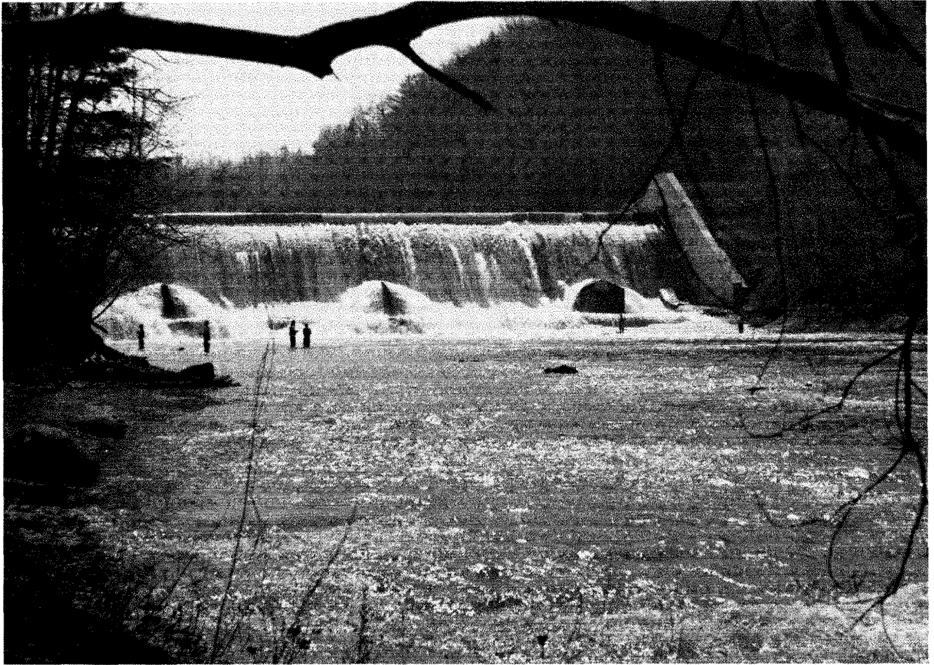
Springville Dam on Cattaraugus Creek
