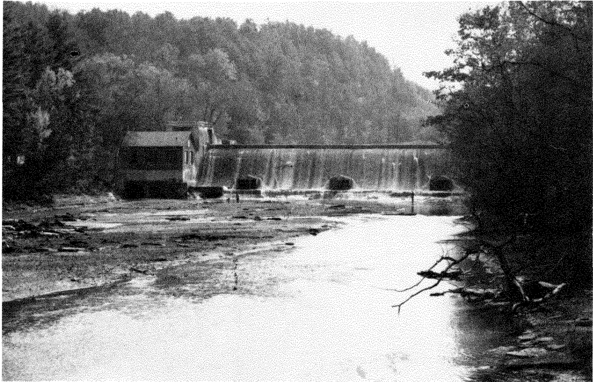
CATTARAUGUS CREEK AT SPRINGVILLE DAM DOWNSTREAM OF THE WVDP
