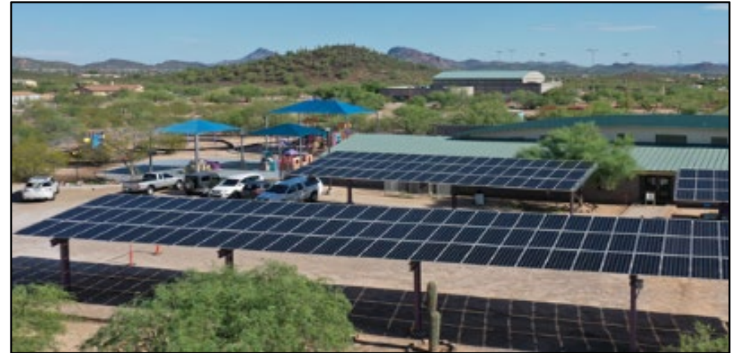
Clockwise from top right: Ute Mountain Ute Tribe (CO) installed a 1-MW solar system (2019); San Xavier Education Building (AZ) installed a 182-kW solar system (2022); and Winnebago Tribe (NE) installed a 23-kW solar system (2016)
