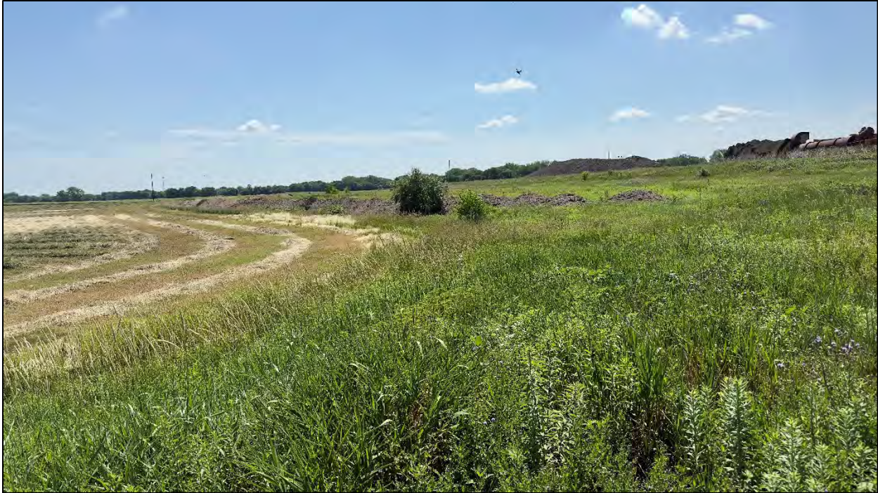
Photograph 5: Southern portion of the Project area view, Southeast
