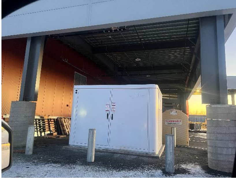
Figure I.21.1 SWS's Electric Vehicle Supply Equipment (EVSE) battery and charger installed by eCamion located at the new Central Transfer Station November 23, 2022. Photo Credit: Kelli Toth
