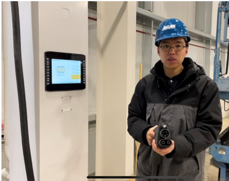
Figure I.21.2 SWS's EVSE charging stations. Members of the team from eCamion were on site to inspect the installation located at the new Central Transfer Station November 23, 2022. Photo Credit: Kelli Toth
