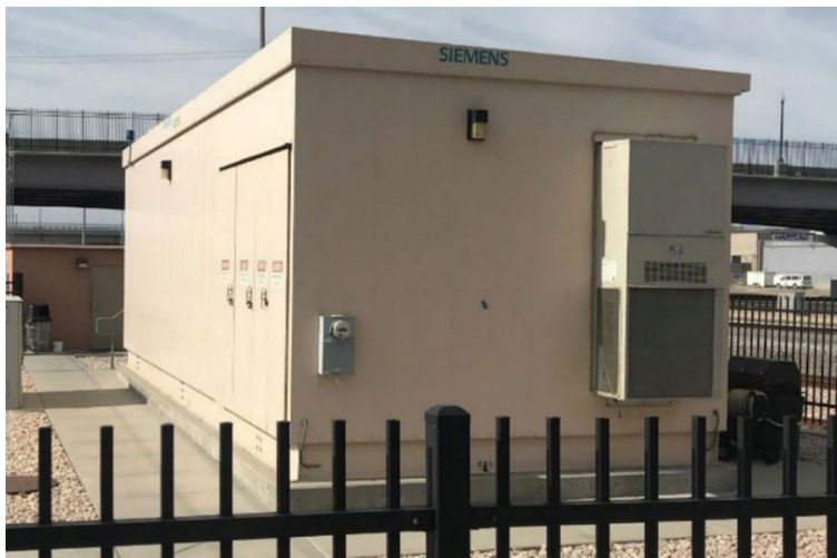
Figure I.26.4 Traction Power Substation (left) and Overhead bus charger (right) (Photo: Utah Transit Authority)
