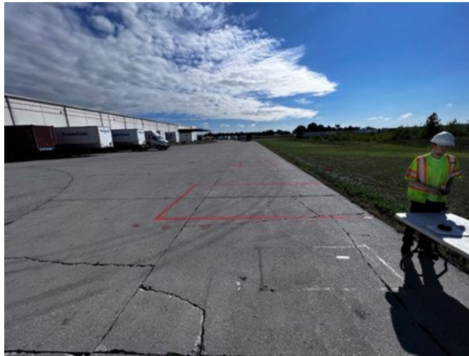
Figure II.1.2.4 Marked the charger location at the site
