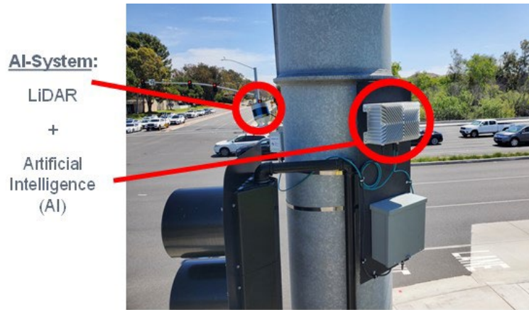
Figure II.1.14.1 Installation of AI-System at intersection of Culver Drive and University Dive.
