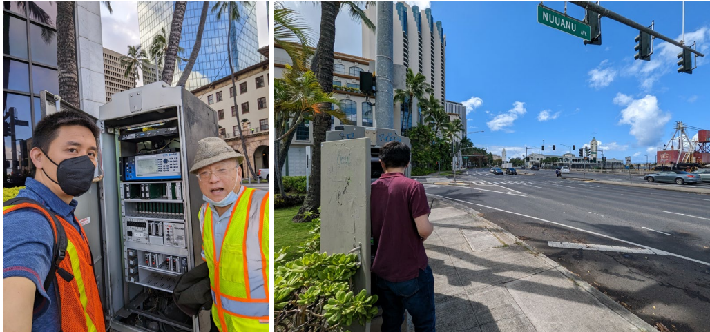
Figure I.3.3.14 Online testing – field observation in April 2023
