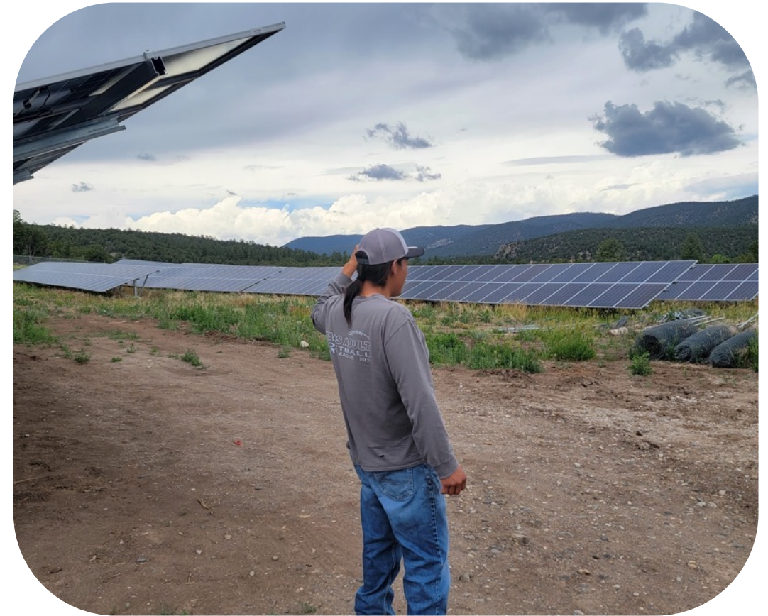
Picuris Pueblo Solar Array – Pictured Celestino – Utilities Technician. Photo by Sherralyn Sneezer
