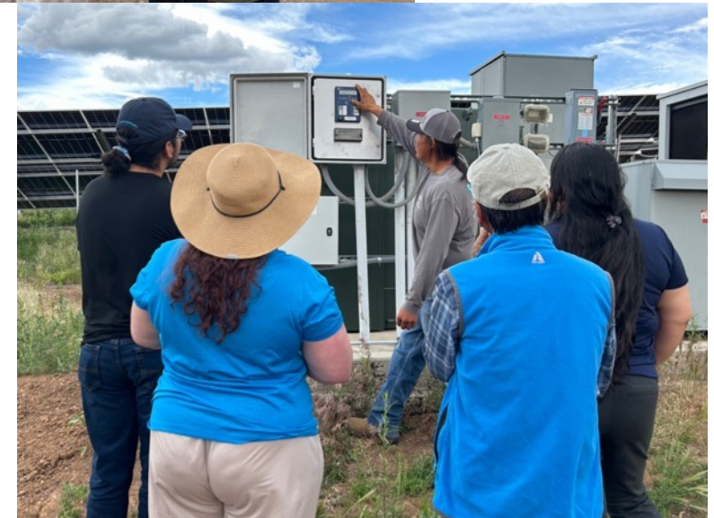
Picuris Pueblo Solar Arrays, Photos by Jennifer Valdez
