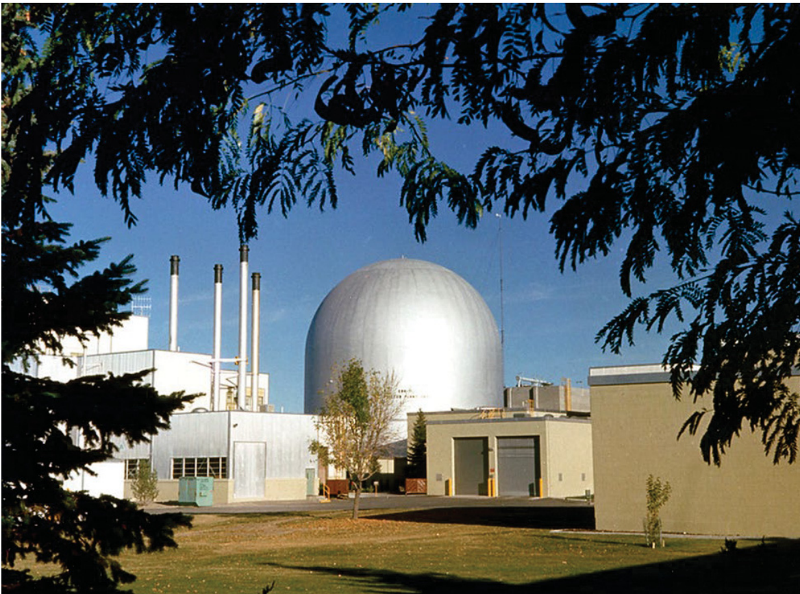
Figure 2. EBR-II reactor plant building in foreground
