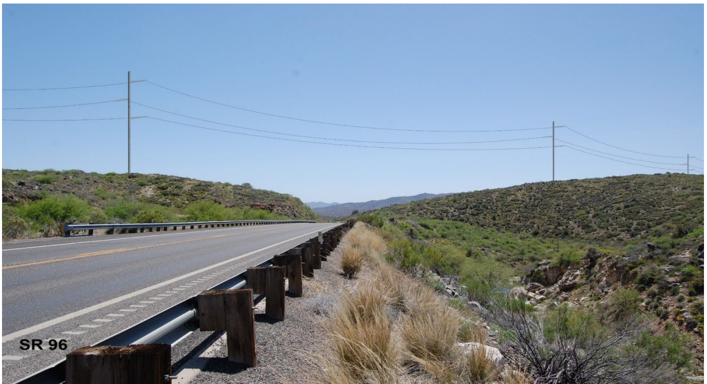
Photo 10. View from Key Observation Point 5 with the proposed Project structures visible.
