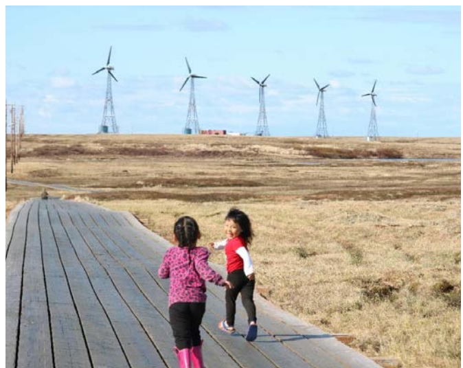
Children run along the boardwalk in the remote village of Kongiganak on Alaska's Yukon-Kuskokwim Delta where wind energy and a battery storage system provide up to 100 percent of the community's electric needs. Photo by Amanda Byrd, Alaska Center for Energy and Power.
