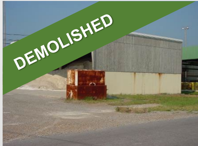
C-732-1 Salt Facility
