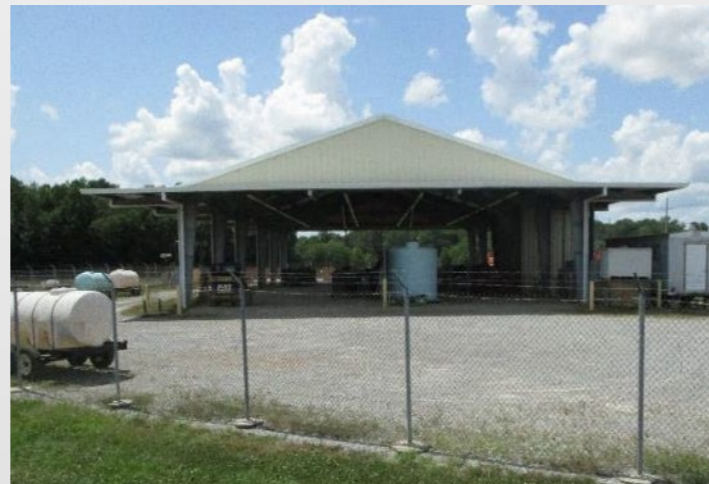
C-752-C Laydown Yard
