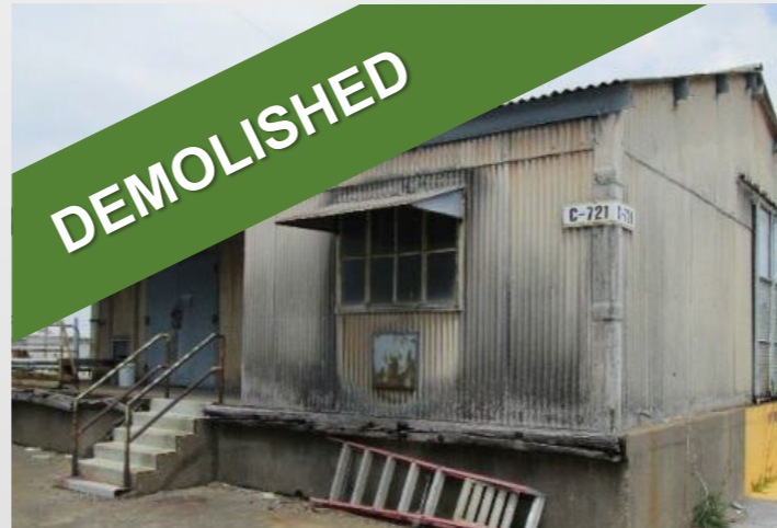
C-721 Gas Manifold Storage
