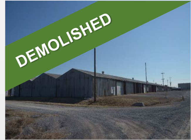
C-746-A North Warehouse
