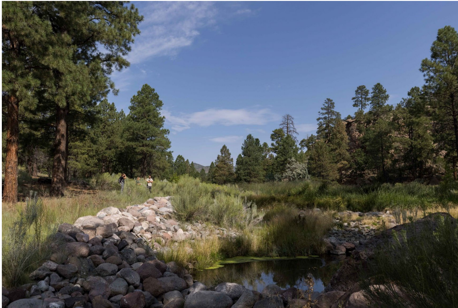
Sandia Canyon storm water control
