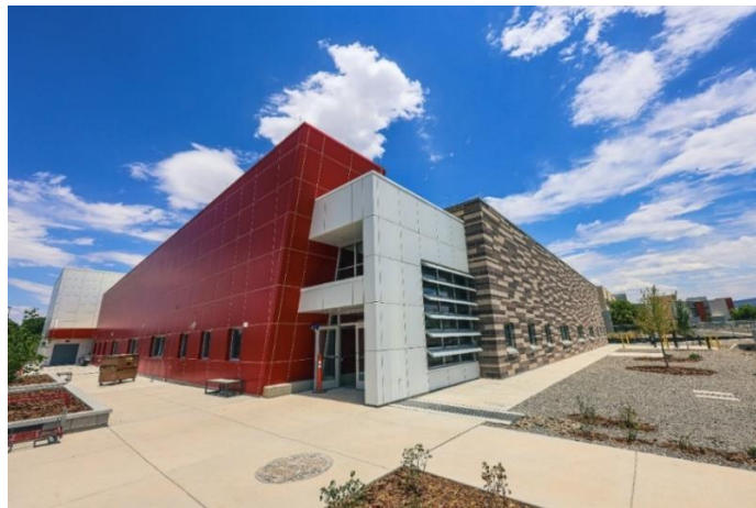
Sandia Emergency Operations Center
