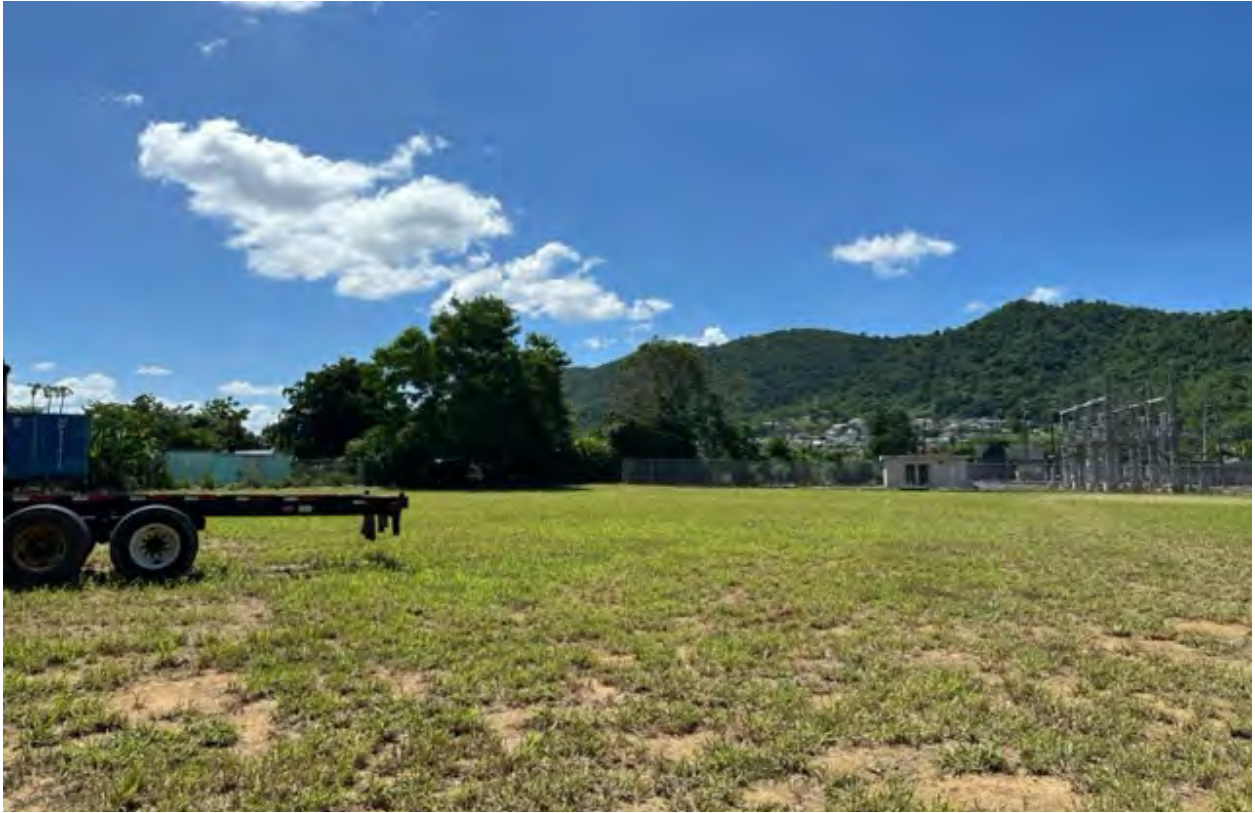
Photo #1 – View toward the northwest at the proposed Caguas BESS site.
