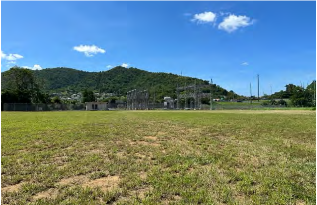
Photo #2 – View toward the north at the proposed Caguas BESS site.
