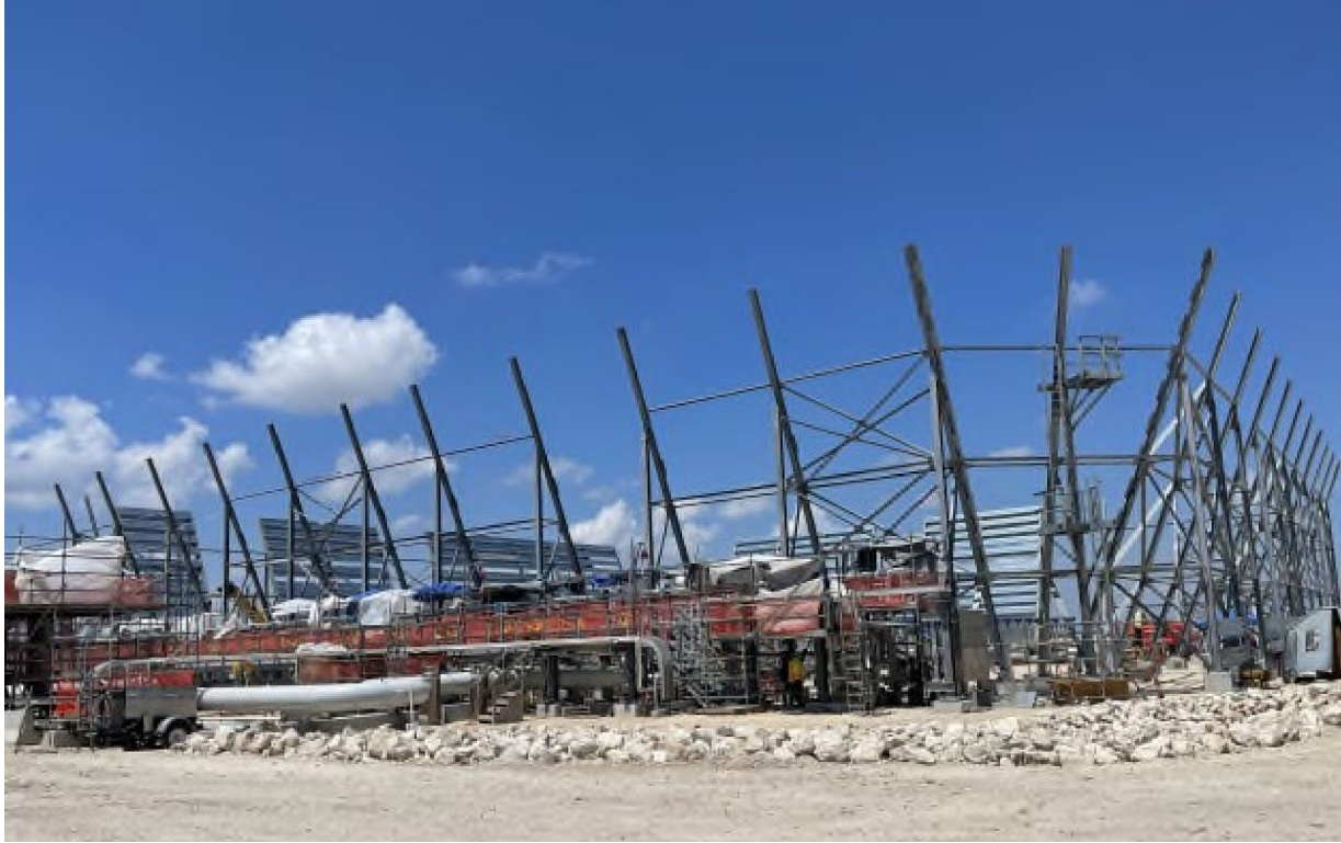
Photo 4: Ground Flare 1 Barrier Erection
