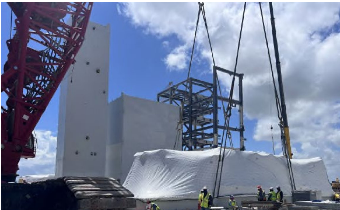
Photo 2: Train 4 Mixed Refrigerant Compressor Set
