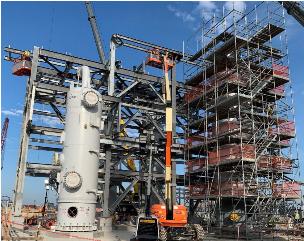
Photo 1: Train 4 Structural Steel
