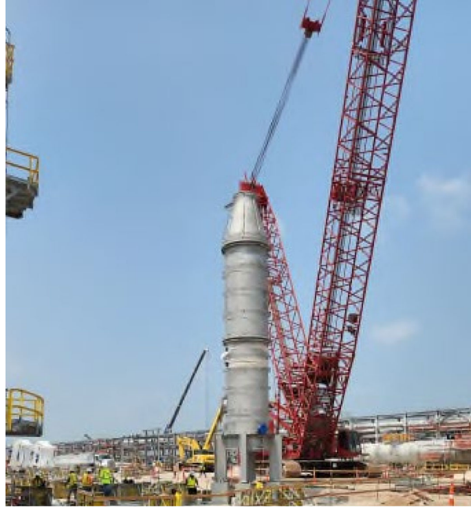
Photo 2: 322M01Train 2 Thermal Oxidizer Setting
