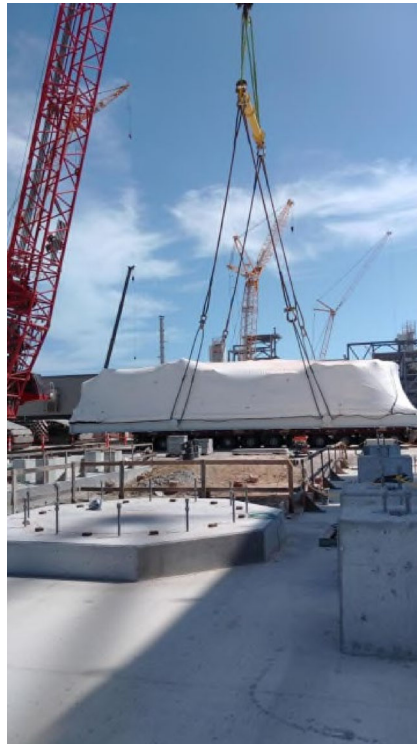
Photo 4: 333A02 Train 3 Refrigeration Compressor Setting
