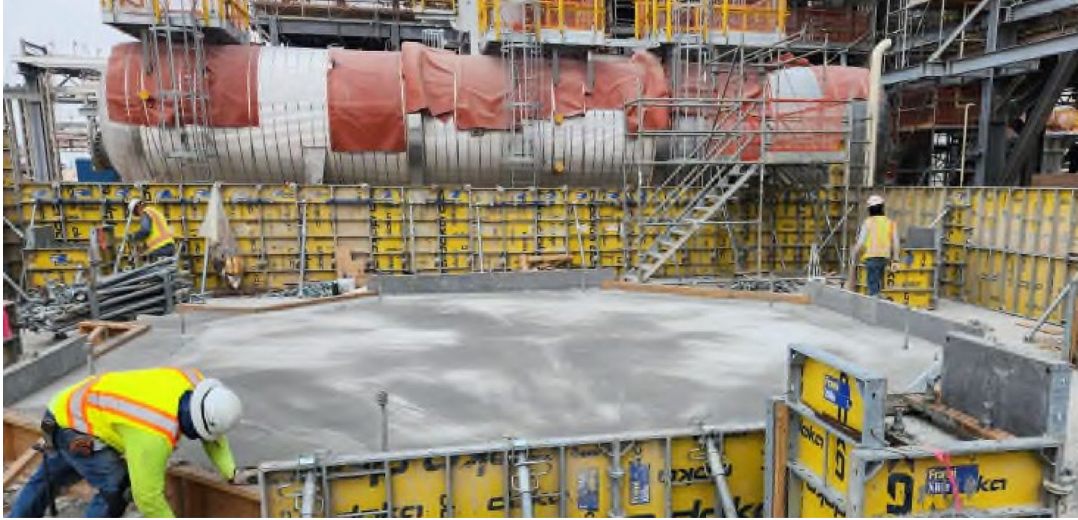
Photo 4: 311L01 Train 1 Amine Tank Foundation
