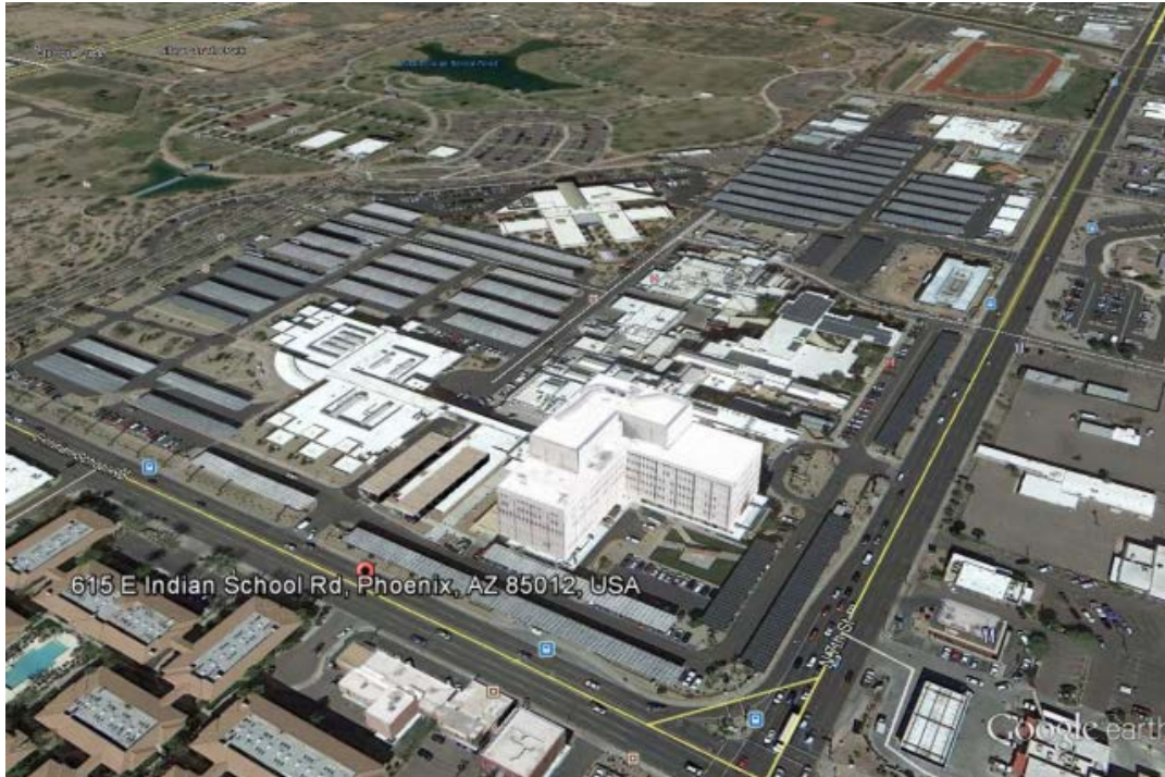
Figure 6. 4.4-MW solar array at Carl T. Hayden VA Medical Center
