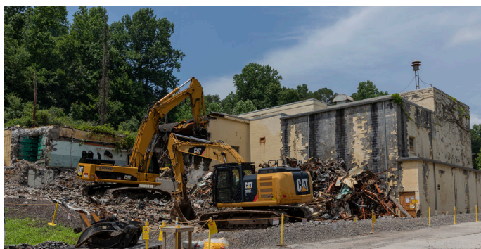
Crews demolish Building 9213
