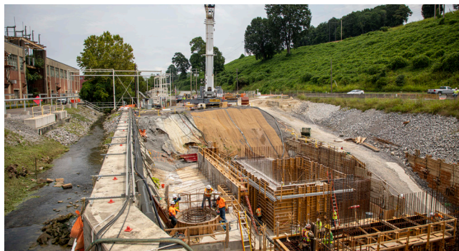
Construction progress on the headworks facility
