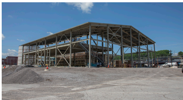
Construction progress on the treatment facility
