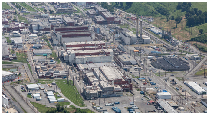
EM is tasked with demolishing numerous excess contaminated facilities, like these, at Y-12
