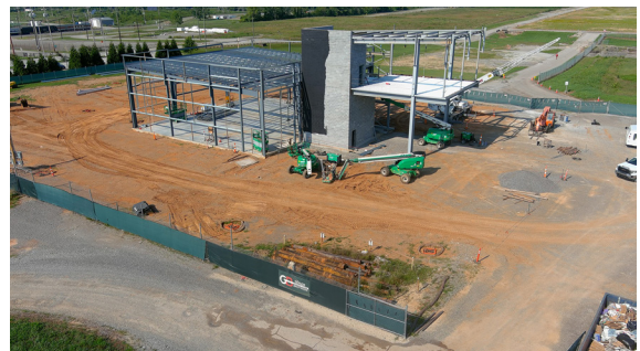
Construction progress on the K-25 Viewing Platform
