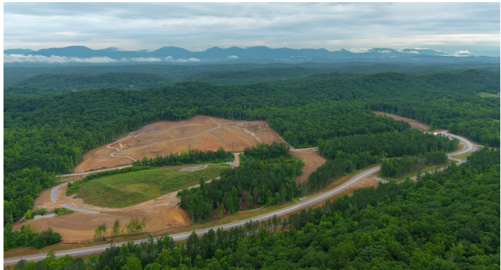
Early site prep is complete, and the future footprint of EMDF is taking shape
