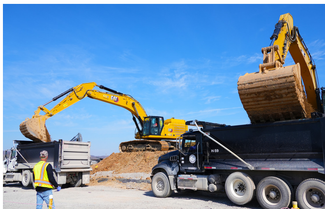
Crews excavated 500,000 cubic yards of soil at ETPP
