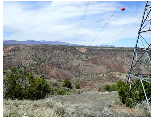
The existing electrical transmission line crossing the Rio Grande to LANL (called the Reeves Line). The proposed path forward would cross at the same location.
