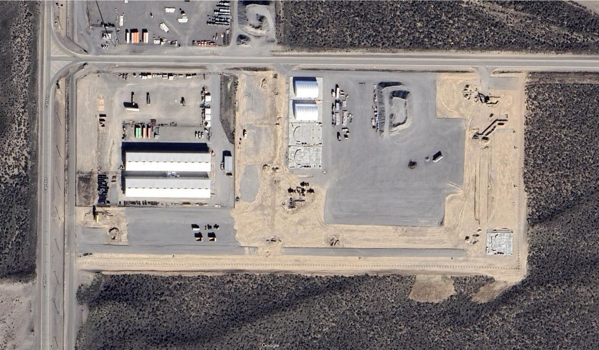
Figure 8. Aerial View of WTP Equipment and Materials Laydown Area at Intersection of Canton Avenue and WTP Loop Road in 200 East Area
