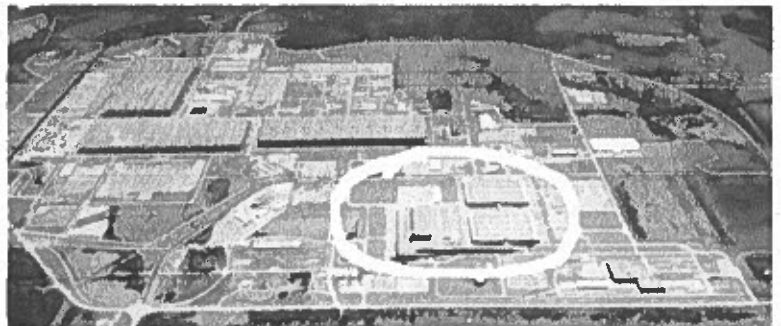
The Portsmouth Nuclear Site with Centrus buildings circled.
