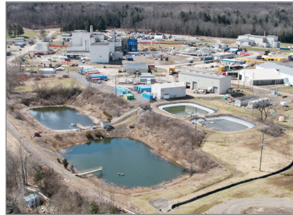
Controlled SPDES discharges occur from the lagoon system
