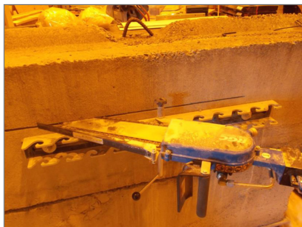
Diamond wire saw (used with misting)
