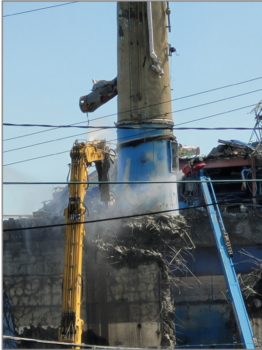
MPPB stack base deconstruction in July 2023
