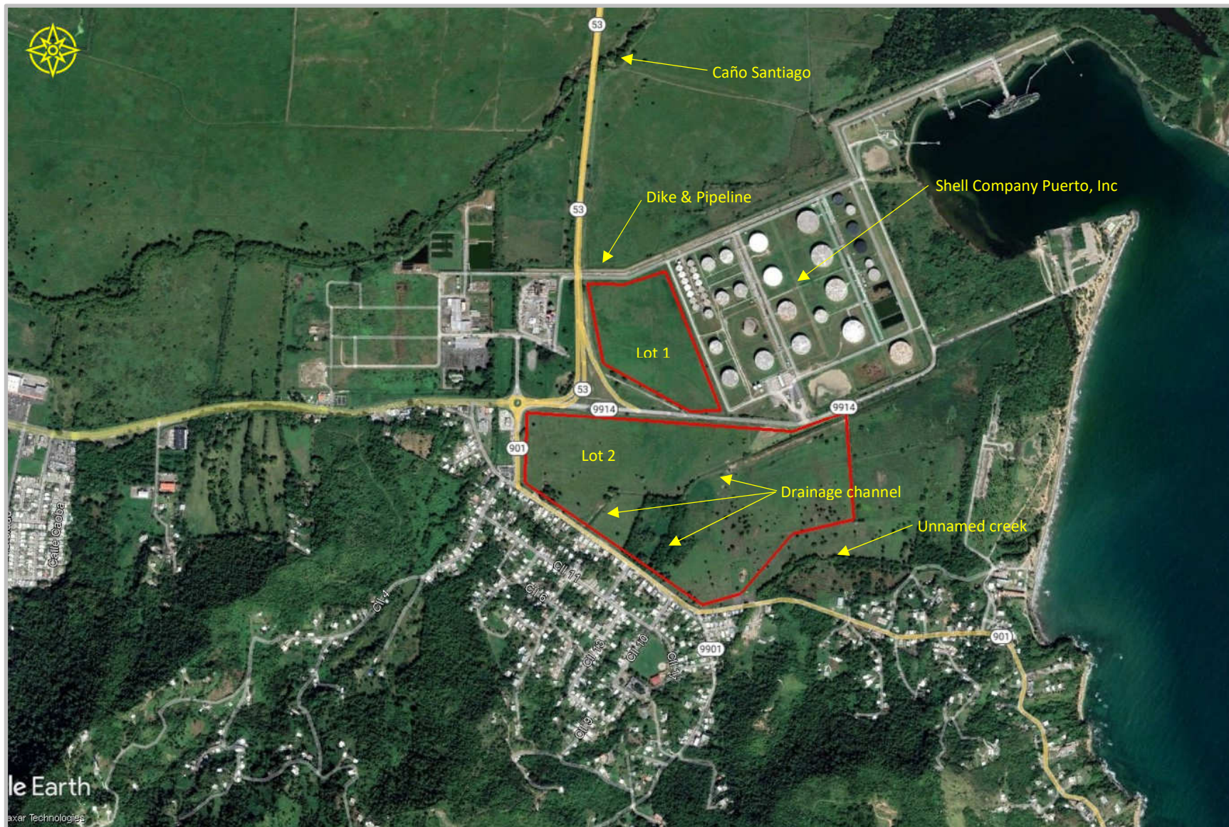
FIGURE 2. Aerial Image (Google Earth; Date: 12/2021) shows the project location, Not to Scale.
