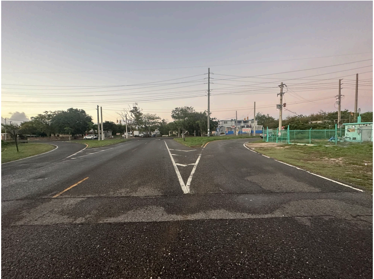
Photo 4 Southbound Approach - Intersection 1
