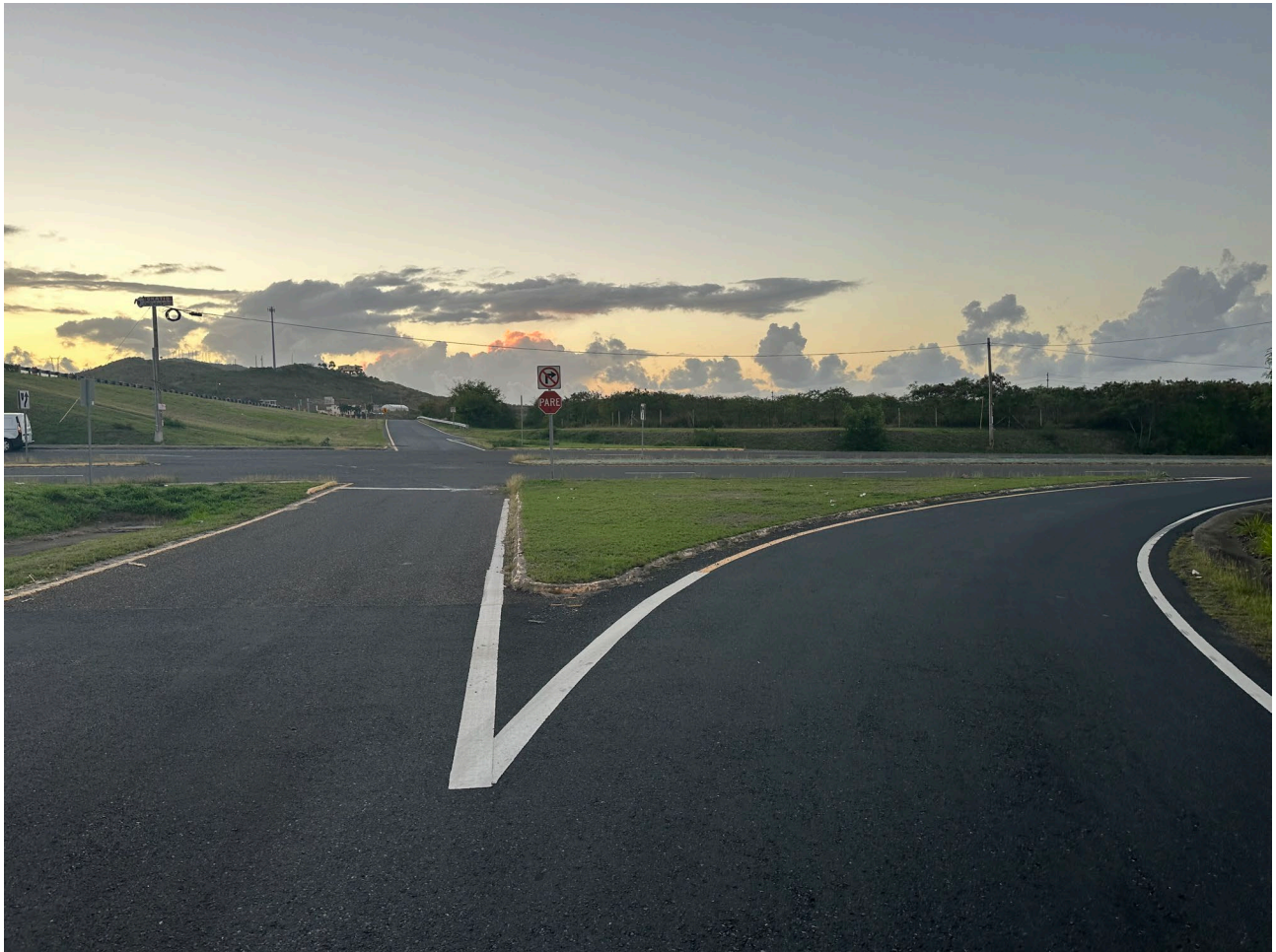
Photo 6 Eastbound Approach - Intersection 2
