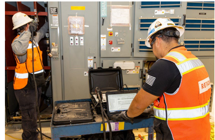
Above: SSCVS large diameter duct work. Below: testing electrical circuits during SSCVS commissioning.
