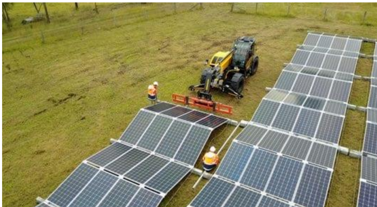
Figure 8. 5B Maverick Modular Structure
