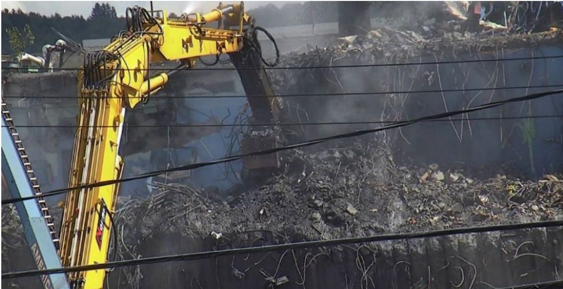
Sample Storage Cell Demolition and Shield Window Removal
