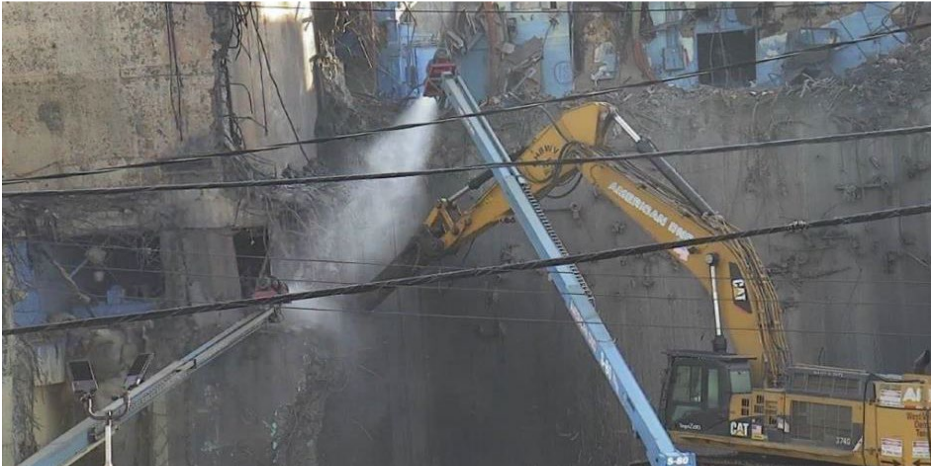
Deconstruction of the Chemical Process Cell North Wall
