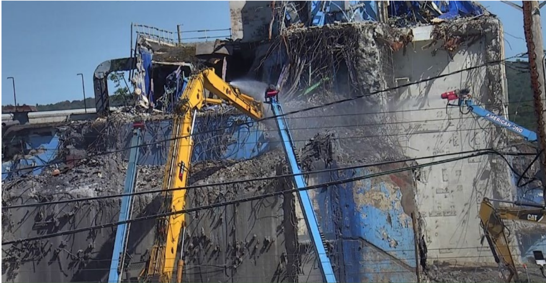
Hot Cell Demo & Shield Door Removal
