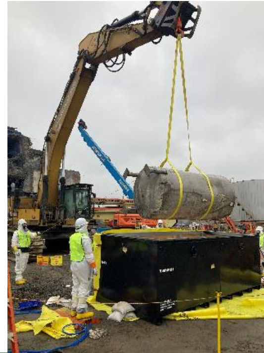
Liquid Waste Cell tanks removed, and one being loaded
