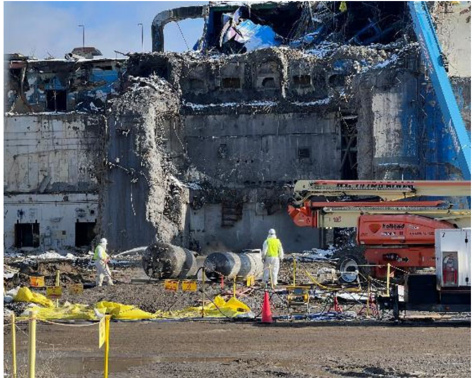
Liquid Waste Cell Tank 3D-2 and 7D-14 removed from Main Plant and prepared for loading
