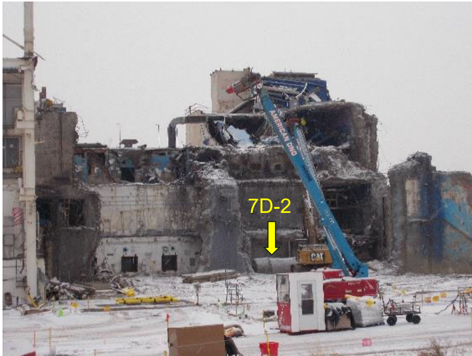
Liquid Waste Cell tank removal (7D-2)
