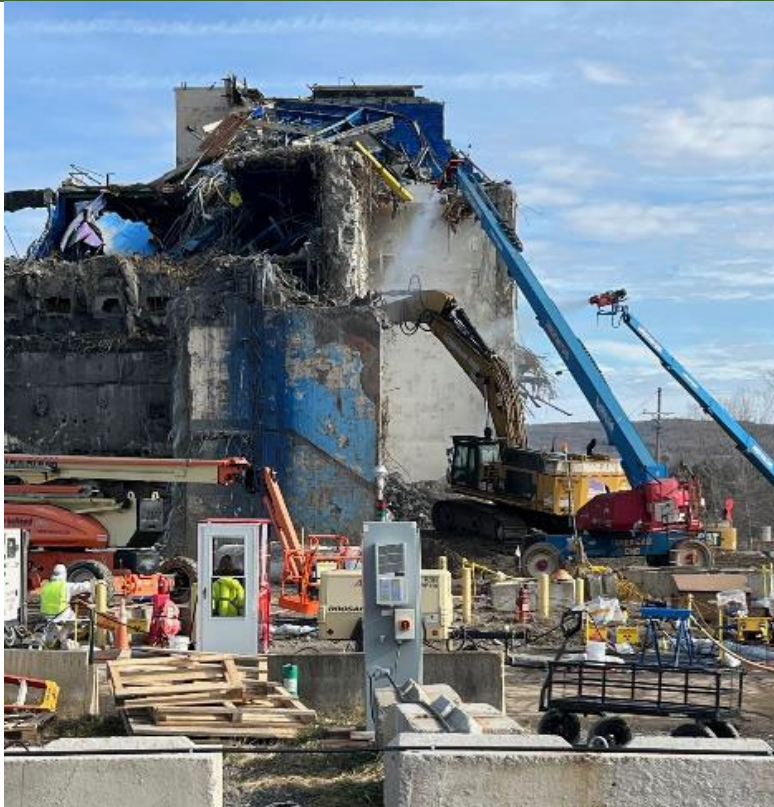
Deconstruction of Extraction Cell #1 north wall
