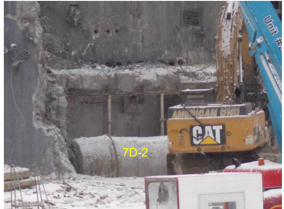
Liquid Waste Cell tank removal (7D-2)
