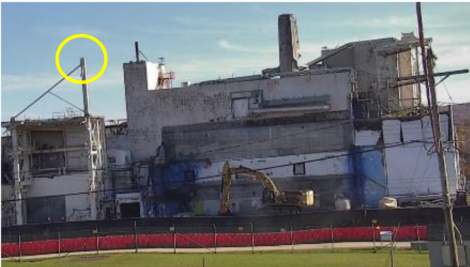
Main Plant west wall before deconstruction (June 2022)
