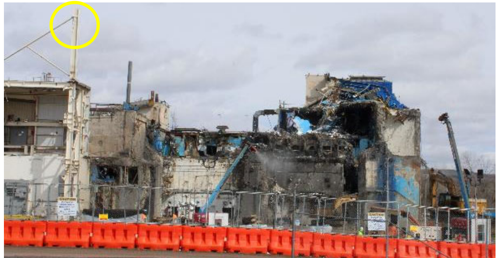
Main Plant west wall (March 2024)
