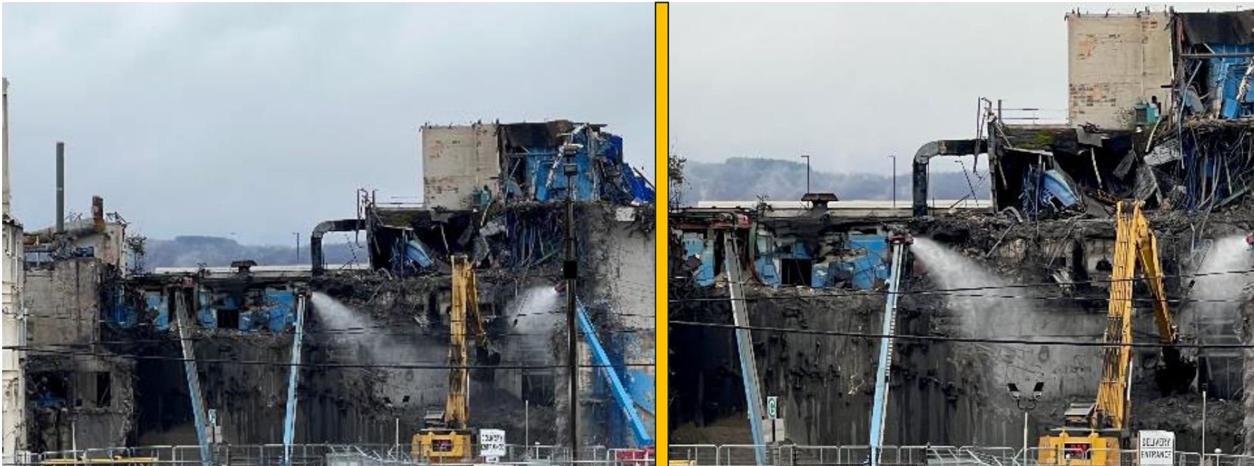
Hot Cell deconstruction
