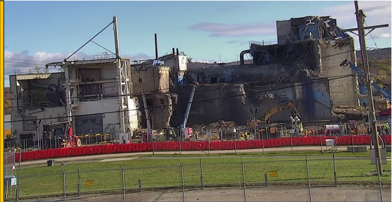
Main Plant West Wall After Deconstruction (October 2023)
