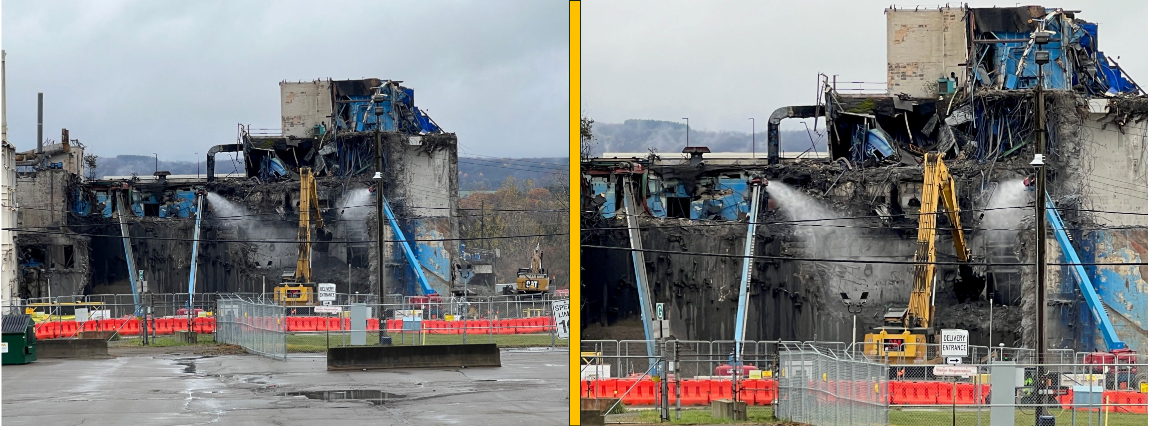
Hot Cell Deconstruction
