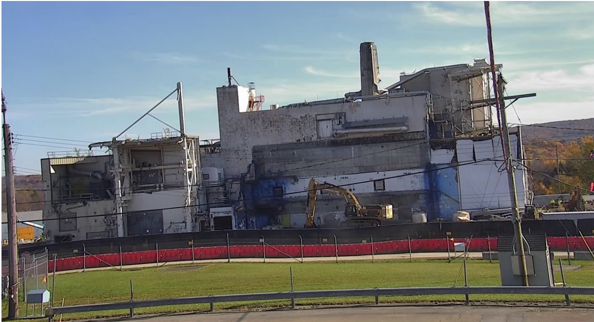
Main Plant West Wall Before Deconstruction (June 2022)
