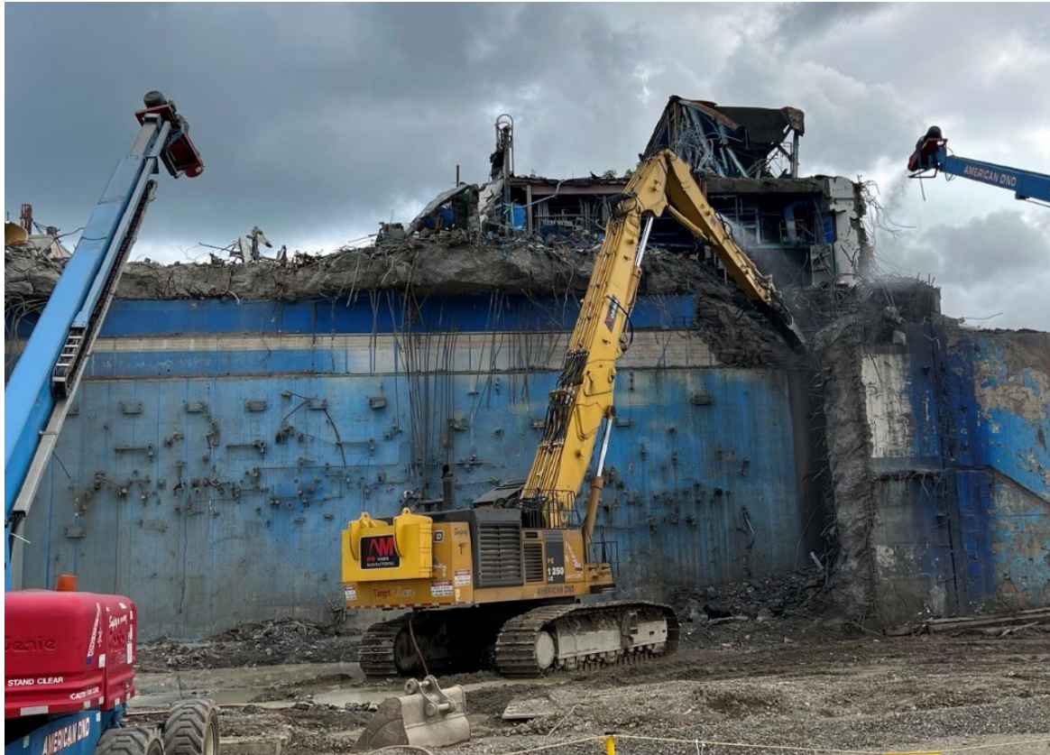
Chemical Process Cell Upper East Wall Removal
