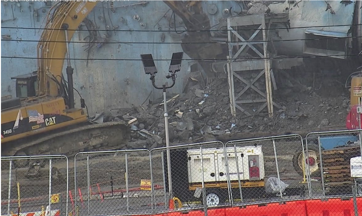
Chemical Process Cell Storage Rack Final Removal and Size-Reduction of Ventilation Stack
