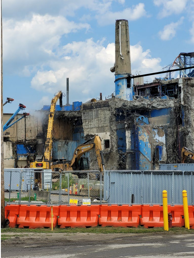
Deconstruction of the Remaining Section of the MPPB Ventilation Stack
