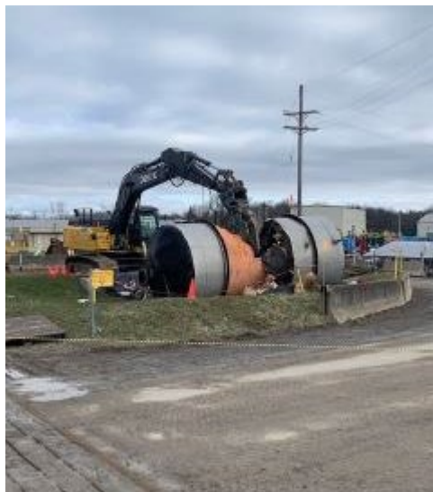
Utility Room Diesel Tank Removal
