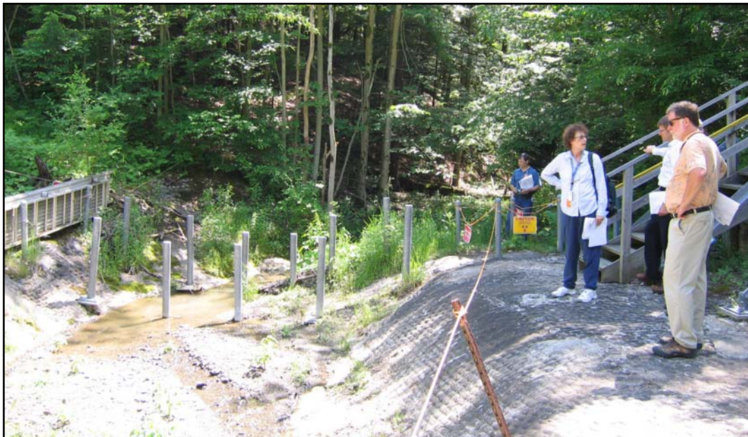
Figure 5-11. Franks Creek Looking Upstream (2008 WVDP photo)
