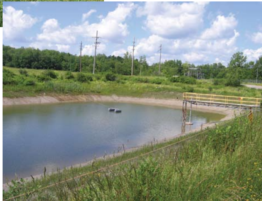
Lagoon 3. Storage Basin for Treated Wastewater Awaiting Discharge to Erdman Brook through the State Pollutant Discharge Elimination System (SPDES) - Permitted Discharge.
