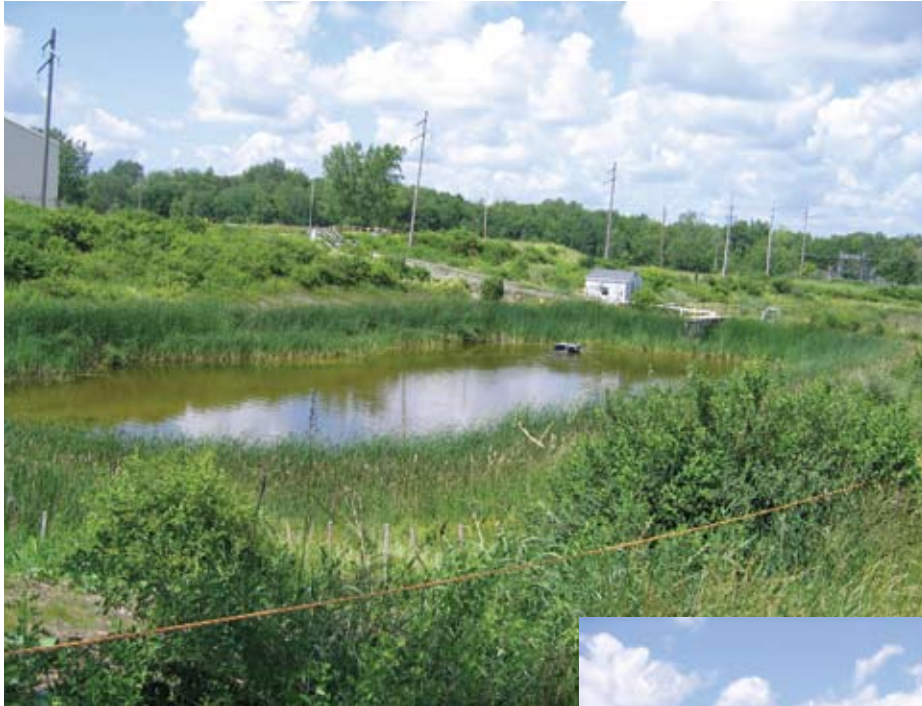
Lagoon 2. Storage Basin for Low-level Radioactive Wastewater Prior to Treatment.
