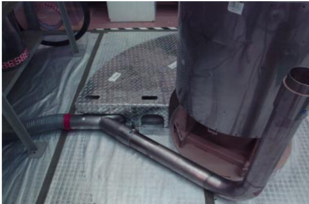
Exhibit 4-1: Ventilation Ductwork for Close Capture System
