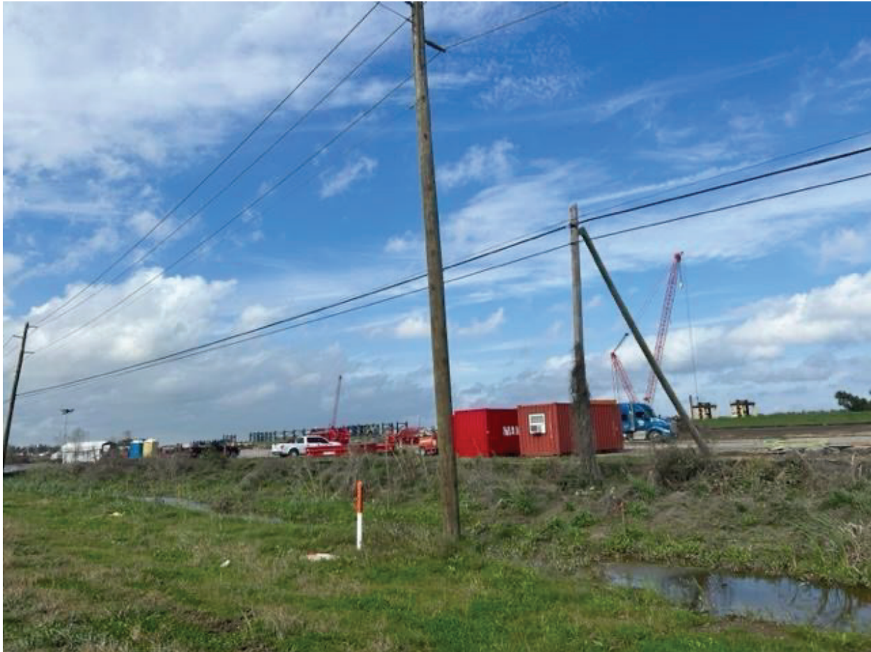
Figure 6.6. Construction Site of Venture Global in Plaquemines Parish
