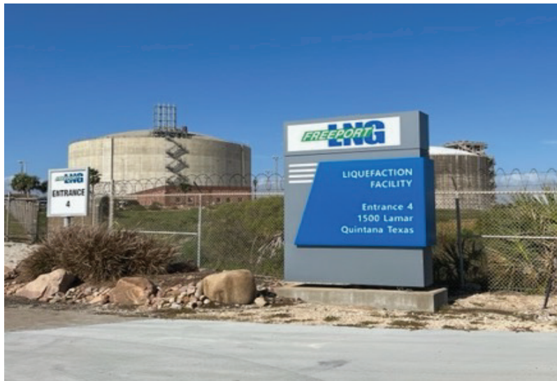
Figure 6.1. Storage Tanks at Freeport LNG
