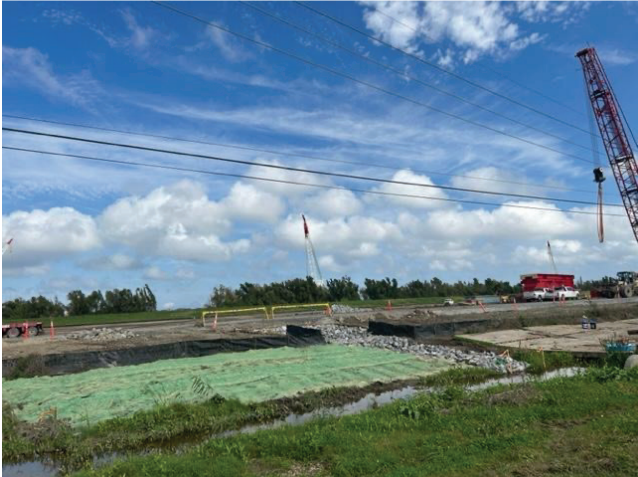
Figure 6.7. Another View of Construction at Venture Global LNG’s Site
