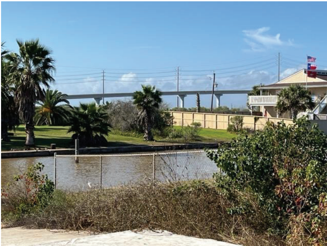
Figure 6.4. Bridge Pictured Is the Only Evacuation from Quintana Island to Freeport
