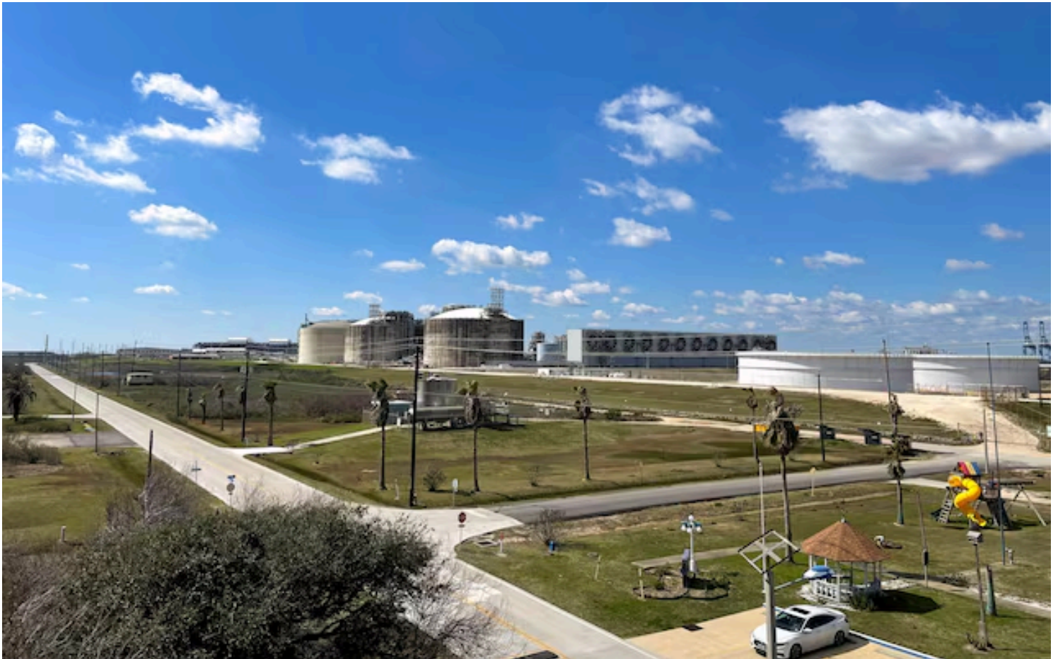
Storage tanks and gas-chilling units are seen at Freeport LNG, the second largest exporter of U.S. liquified natural gas, near Freeport, Texas, U.S., February 11, 2023. Reuters/Arathy... Purchase Licensing Rights Read more
