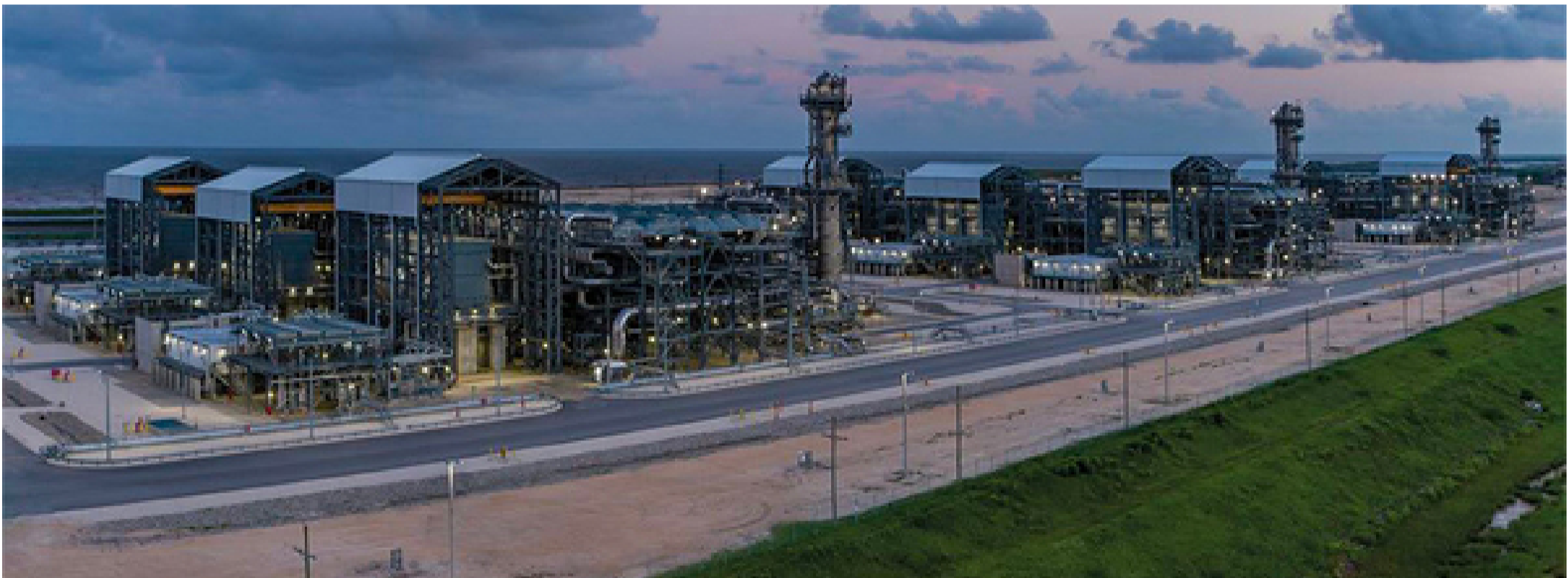
The Freeport liquefied natural gas facility in Texas. Freeport LNG via Business Wire
