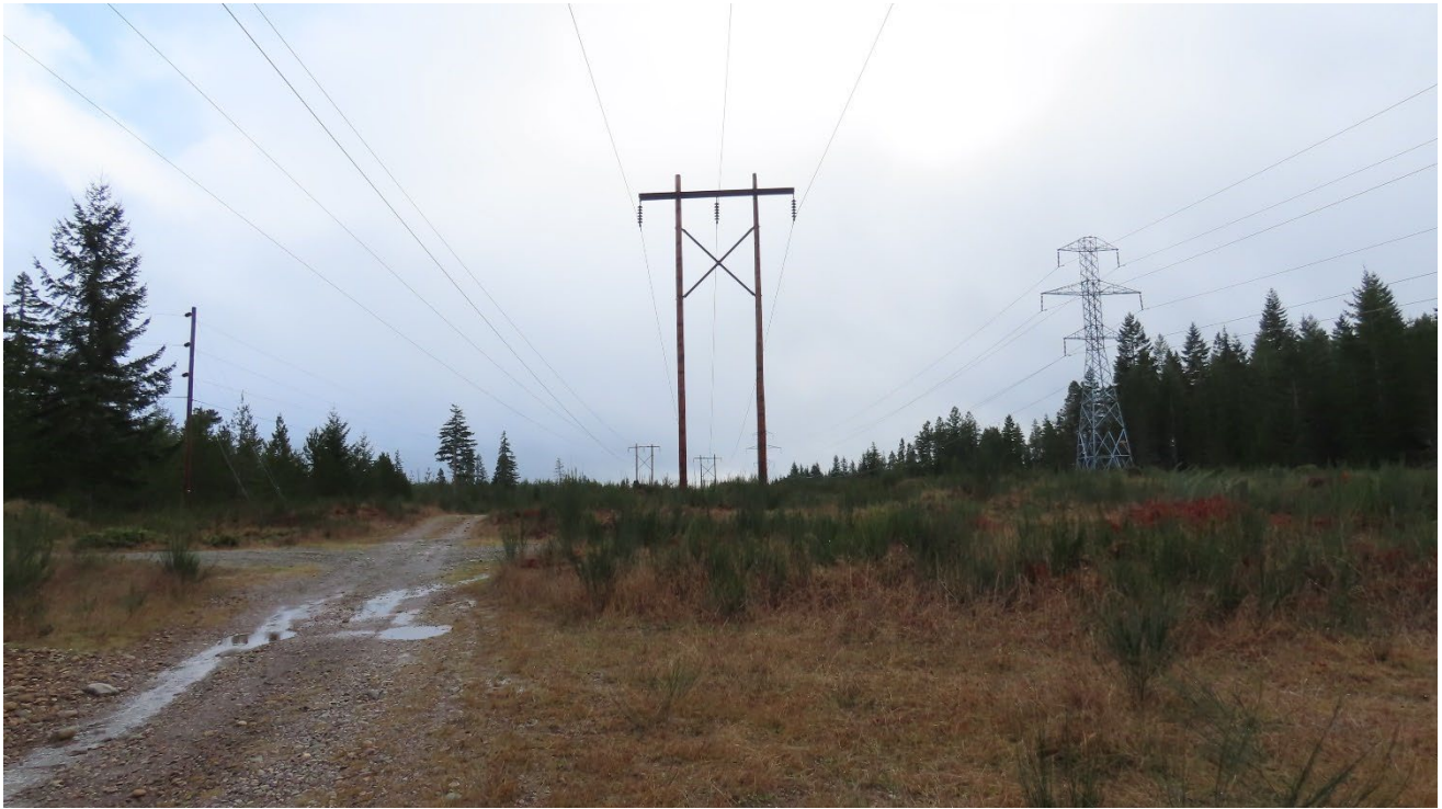
Figure D-1: Existing Two-Pole Wood Structure
