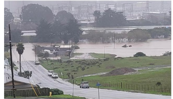
Flooded substation in Morro Bay, CA, January 2023.
