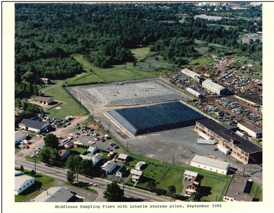
Figure 1. The MSP During Vicinity Property Remediation.
