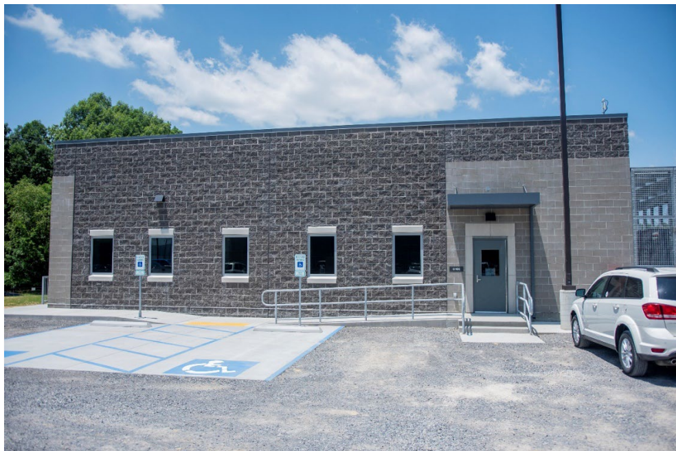
On June 26, 2023, workers completed construction of the new Emergency Operations Center.
