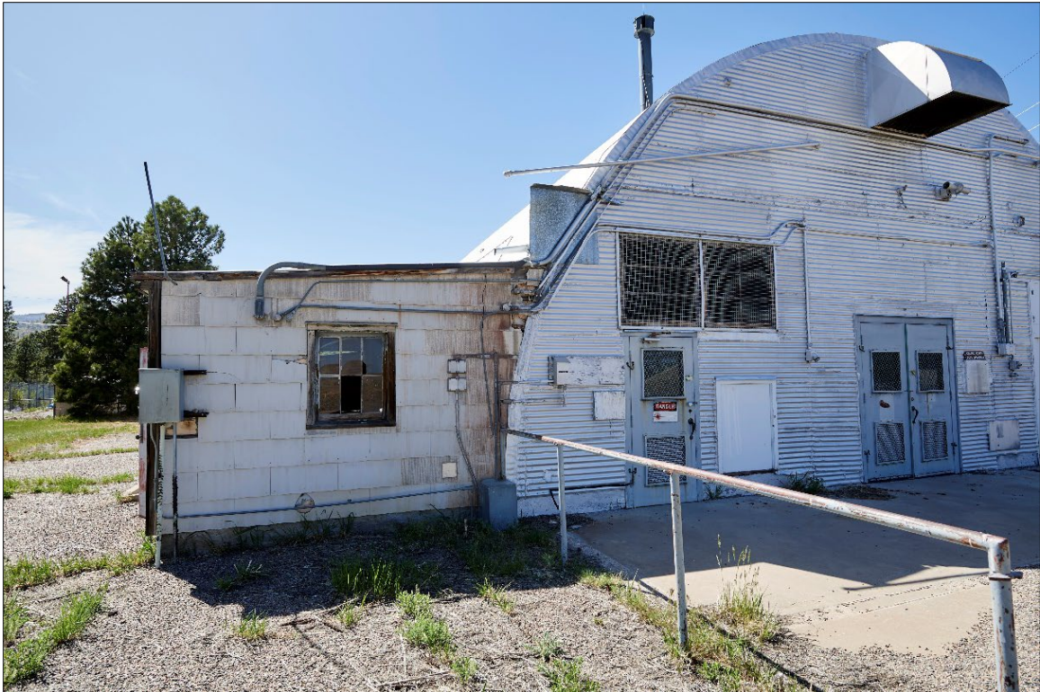
Figure 6. The TA-22-0001 Quonset Hut before the shingle-replacement project began.
