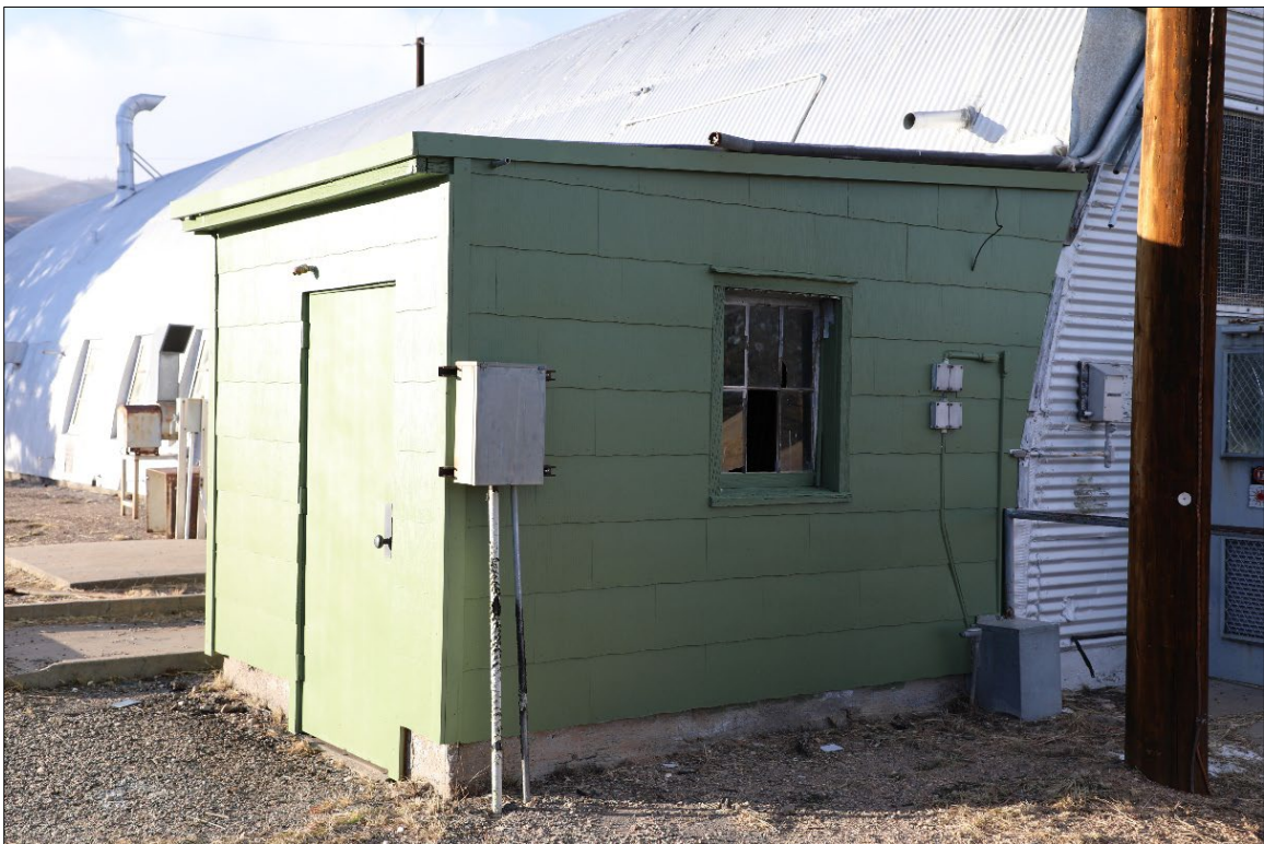
Figure 7. The TA-22-0001 Quonset Hut after the shingle-replacement project was complete.
