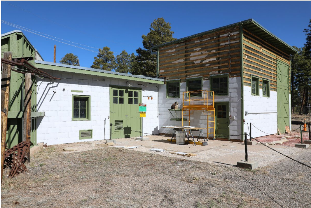
Figure 4. TA-16-0516 and TA-16-0517 (V-Site) during the shingle-replacement project.
