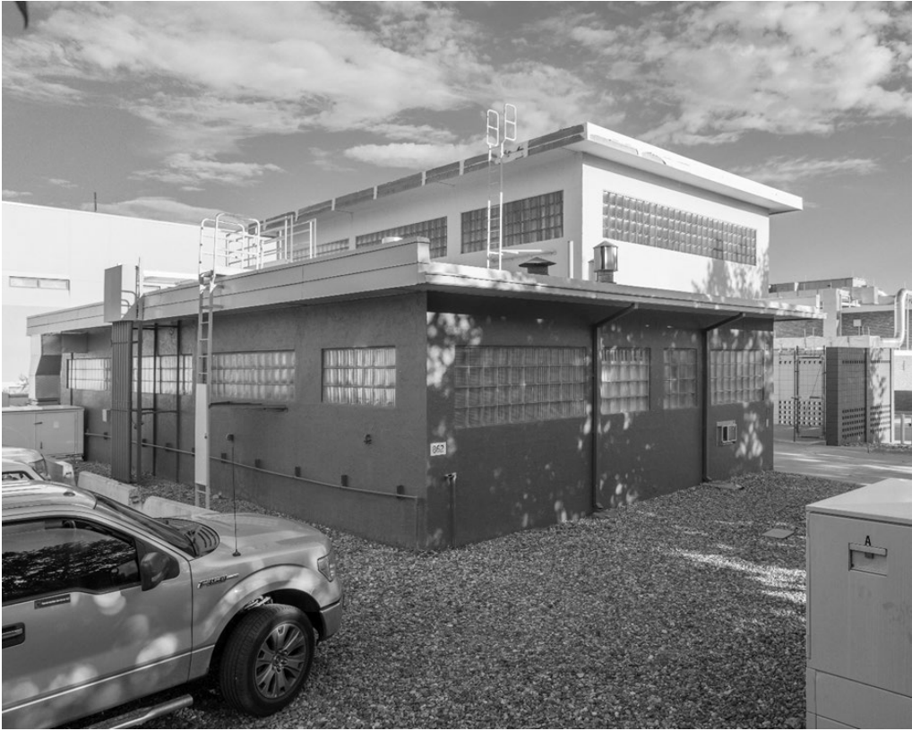
Building 862, south and east sides, featuring rows of glass block windows on low- and high-bay sections
