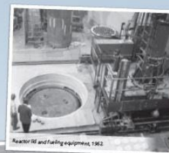
Reactor Vessel and fueling equipment, 1962.
