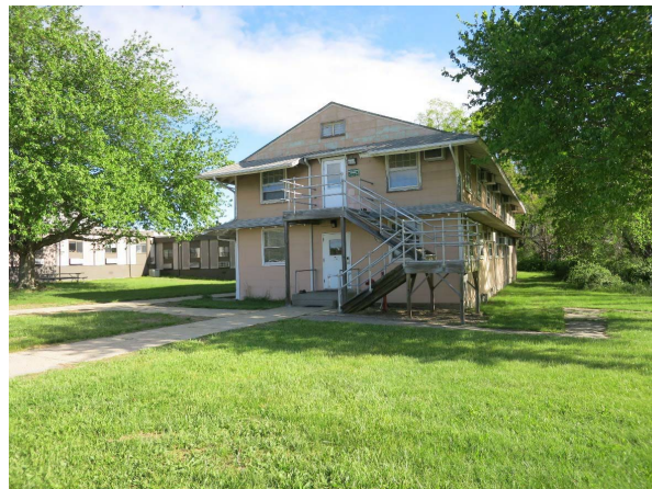
Figure 2: Building 120, representative structure of a Series 700 barracks building dating from 1941.
