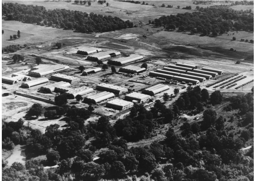
The East Area during Construction in 1948 (Courtesy Argonne National Laboratory Photo Library)
