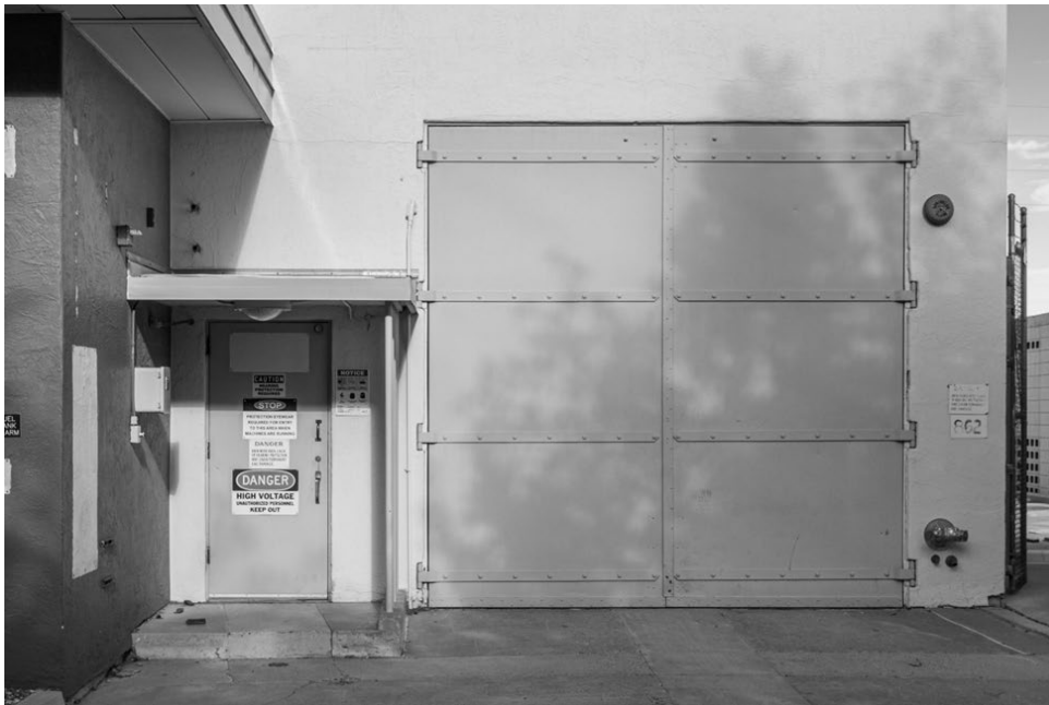
Building 862, east side entrances
