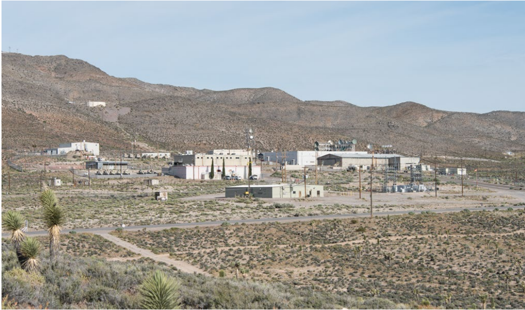
Figure 3: Overview of the Area 6 Control Point Historic District, pictured in 2016 (Remote Sensing Laboratory).
