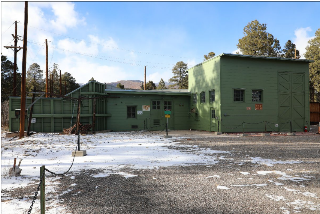
Figure 5. TA-16-0516 and TA-16-0517 (V-Site) after the shingle-replacement project was complete.
