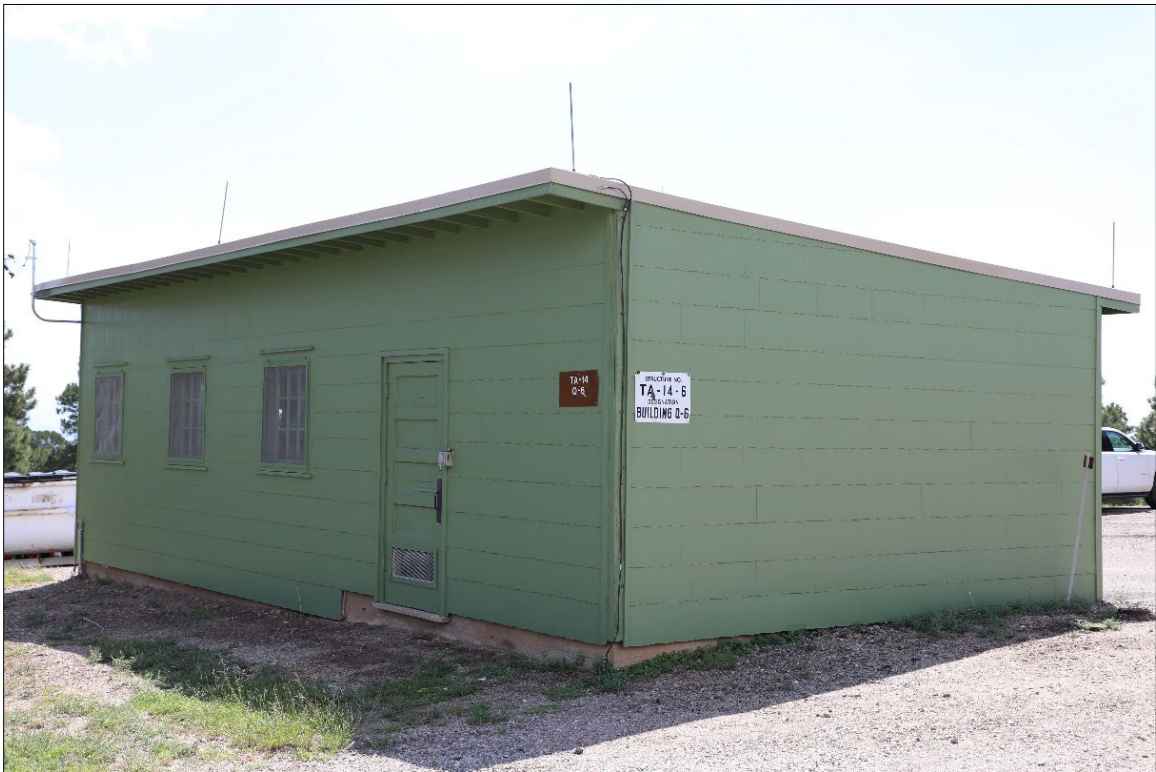
Figure 9. TA-14-0006 (Q-Site) after the shingle-replacement project was complete.
