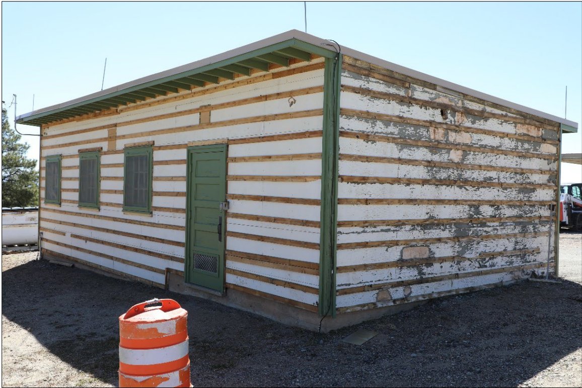
Figure 8. TA-14-0006 (Q-Site) during the shingle-replacement project.
