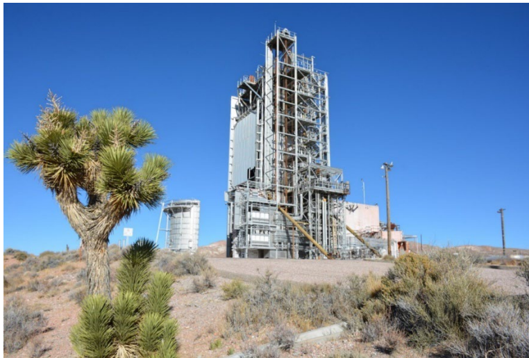
Figure 2: Engine Test Stand 1 at the NRDS (DRI 2021).
