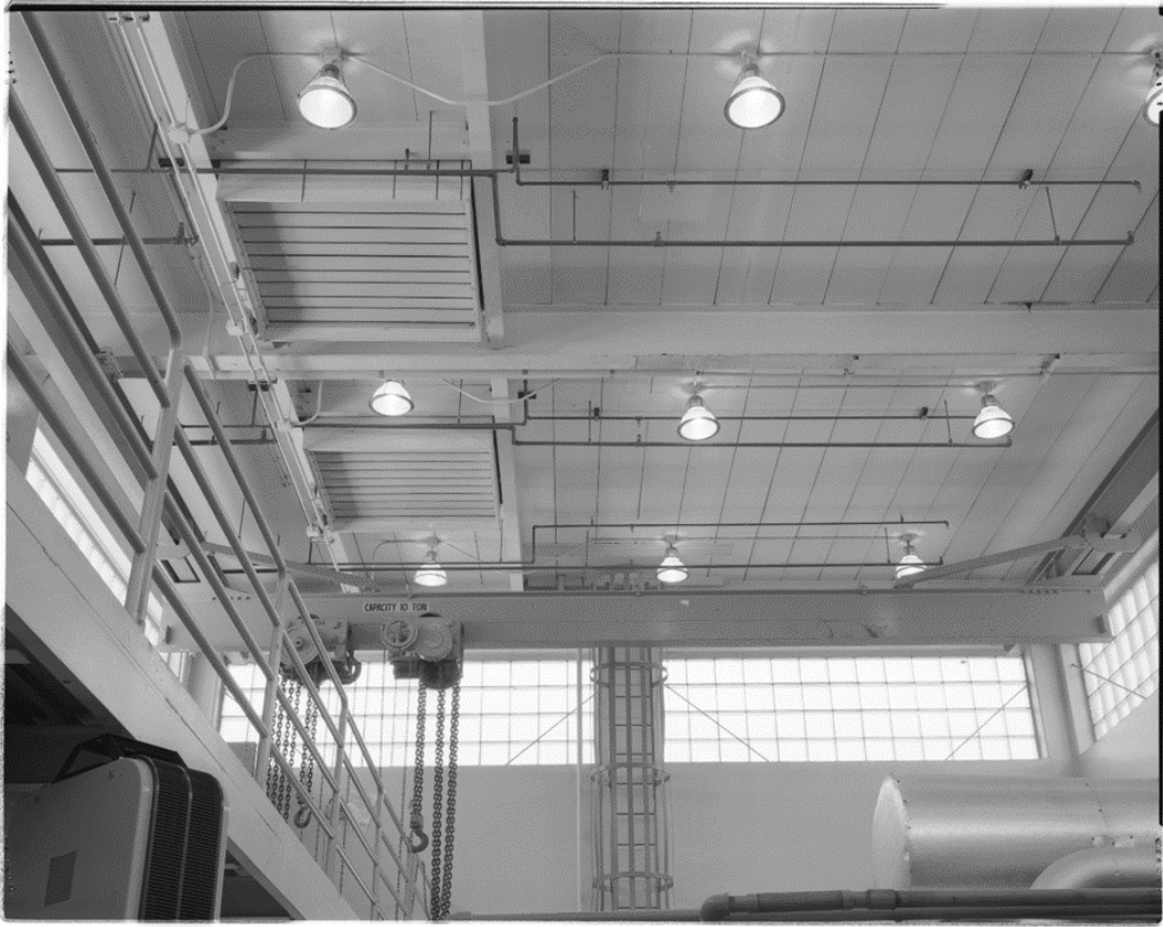
Building 862, interior, high-bay ceiling
