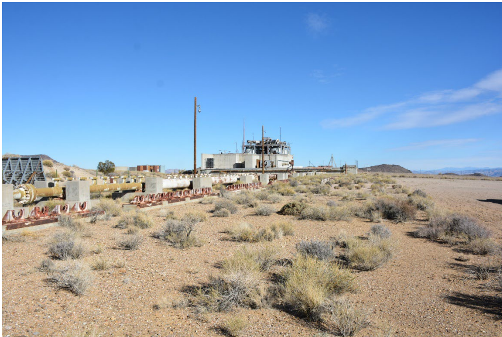
Figure 4: Compressed air rack and pipe remnants with the Pluto Test Bunker in the background. (DRI 2022).
