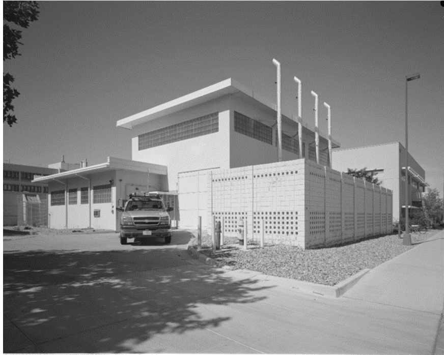
East and south sides, Building 862
