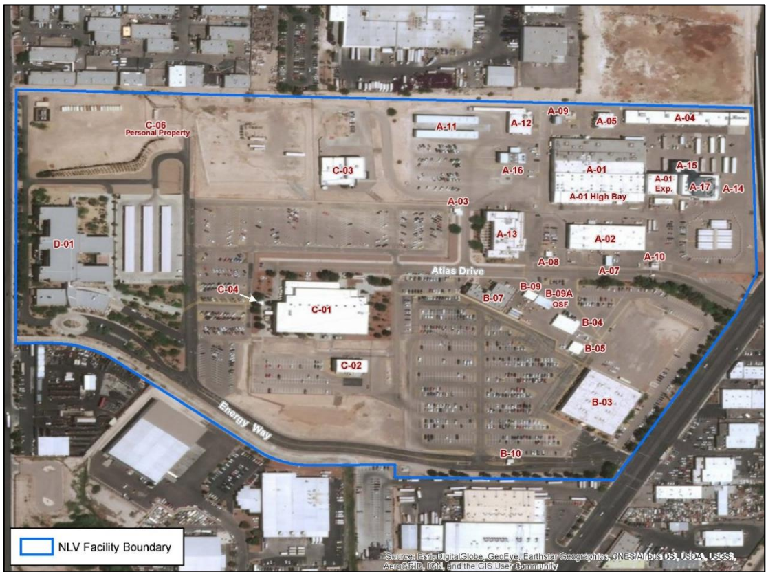
Aerial overview of the NNSA/NFO North Las Vegas facility.
