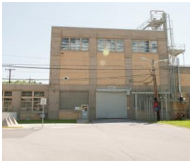
Y-12 National Security Complex Building 9731
