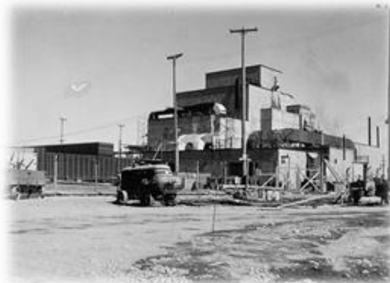
B Reactor (105-B) Under Construction
