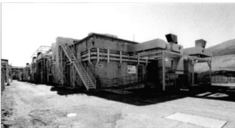
Building 865A, north and east elevations, 2001.
