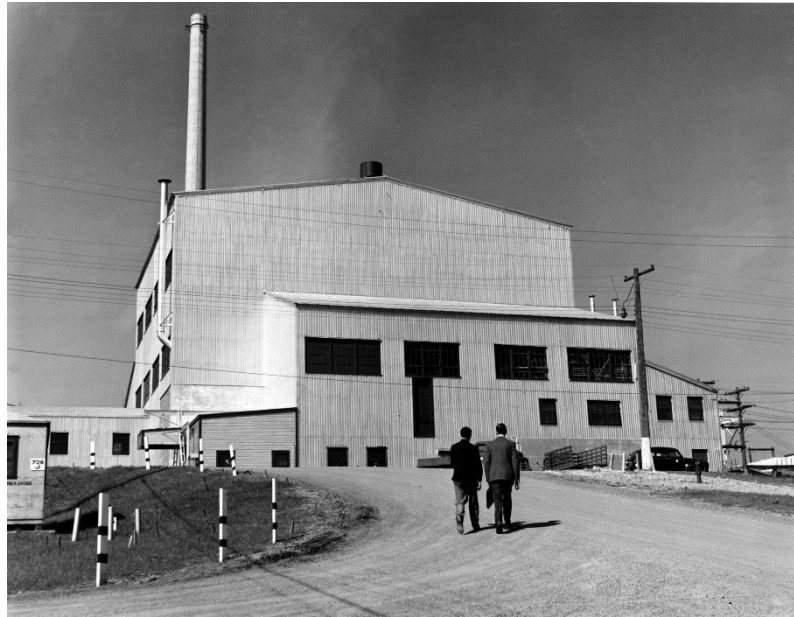
Oak Ridge National Laboratory Graphite Reactor Exterior, 1940s
