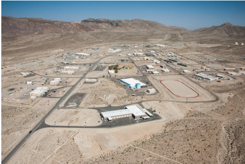
Aerial overview of the town of Mercury, the main base camp at the NNSS.
