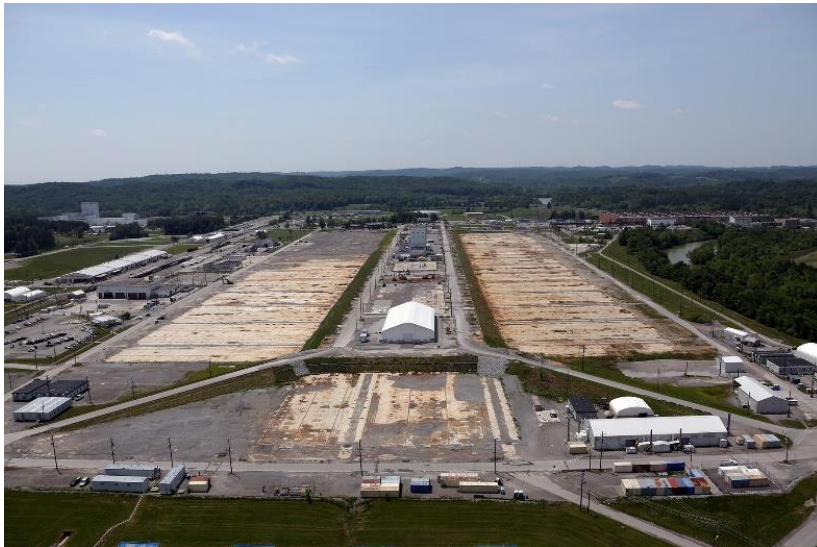
K-25 Building Demolition Footprint
