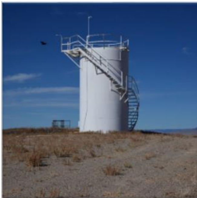
Figure 3: Askania camera tower at TTR.
