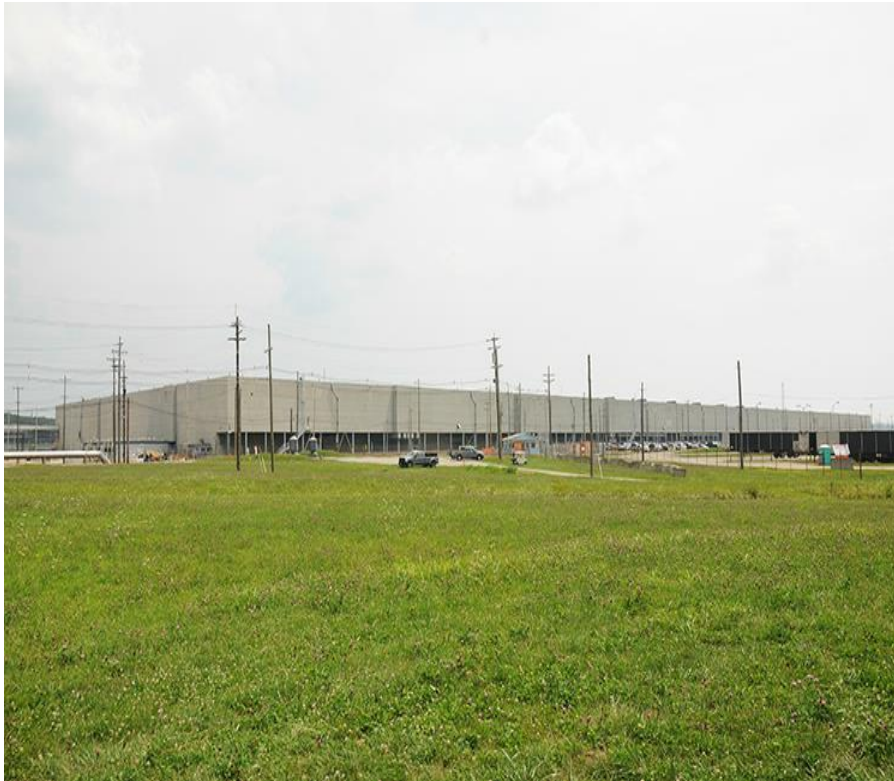
Northwest corner of the X-326 Process Building, facing southeast. Building to be included in the HAER Reports.
