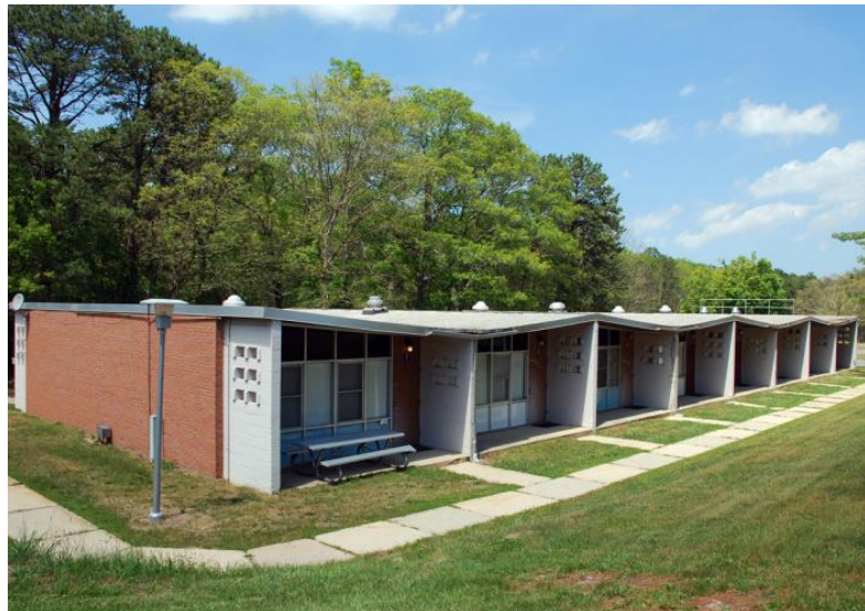
Figure 3: Example of one of four 1960s era efficiency apartment buildings.
