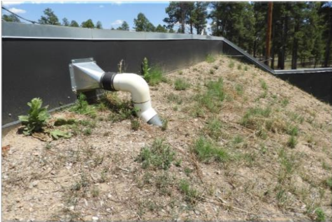
Figure 5: Repaired retaining wall at V-Site.
