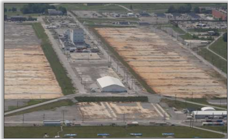
K-25 Building Slab
