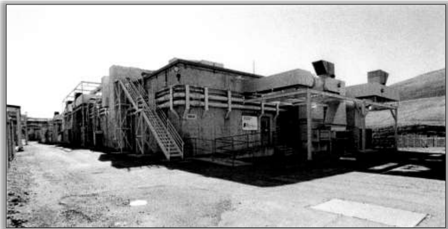
The B865 Complex was built specifically to house the Advanced Test Accelerator (ATA) to investigate the feasibility of directing intense electron beams through atmosphere for use as a defensive weapon.
