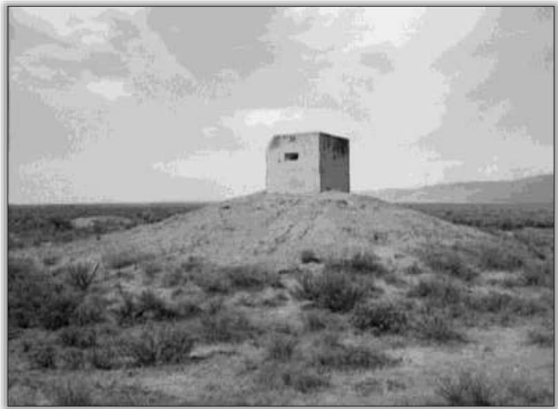
Arco NPG, Mass Detonation Area camera shelter, view looking SW.
