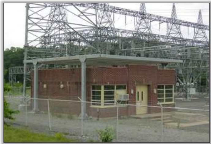
Van Buren Substation Control Building, Van Buren, Arkansas
