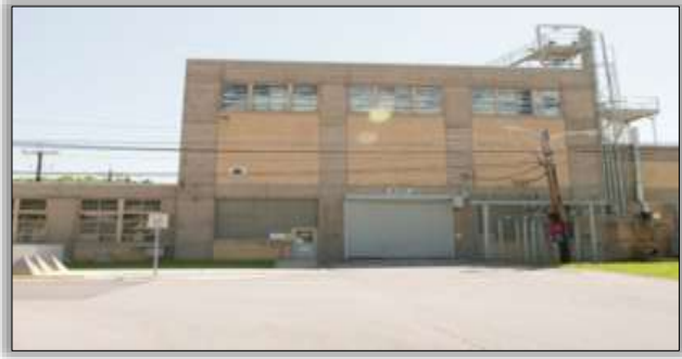
Building 9731 (Pilot Plant)
