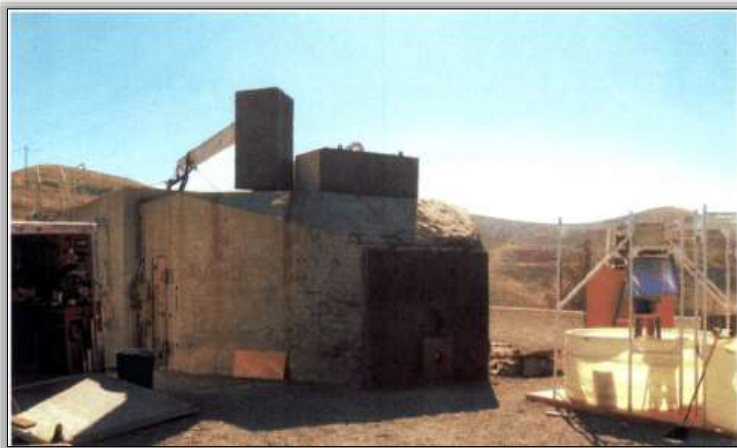
The Firing Facility at B851A was engaged in hydrodynamic testing of non-fissionable nuclear weapons components and devices in support of the LLNL weapons program during the Cold War.
