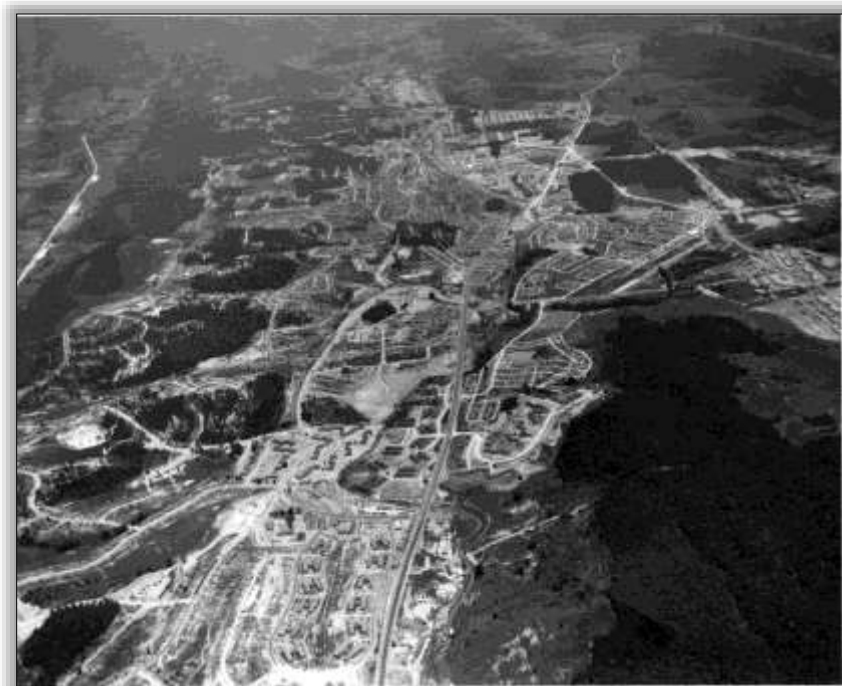
Aerial view of the Oak Ridge Reservation
