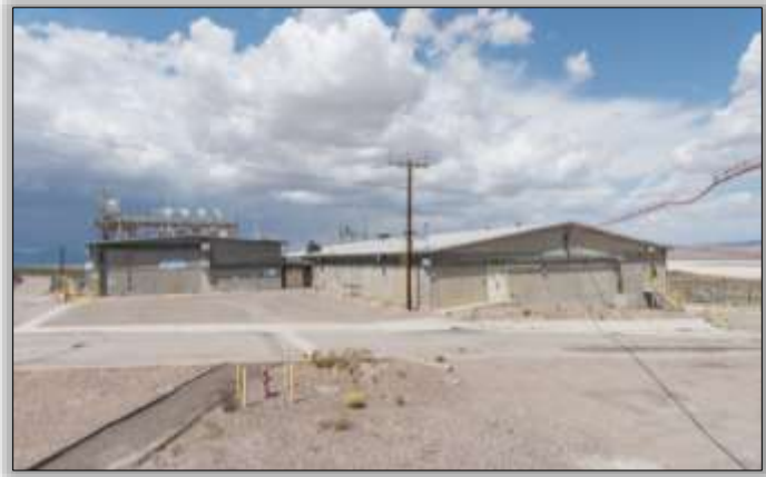
Control Point Building 1 (CP-1)
