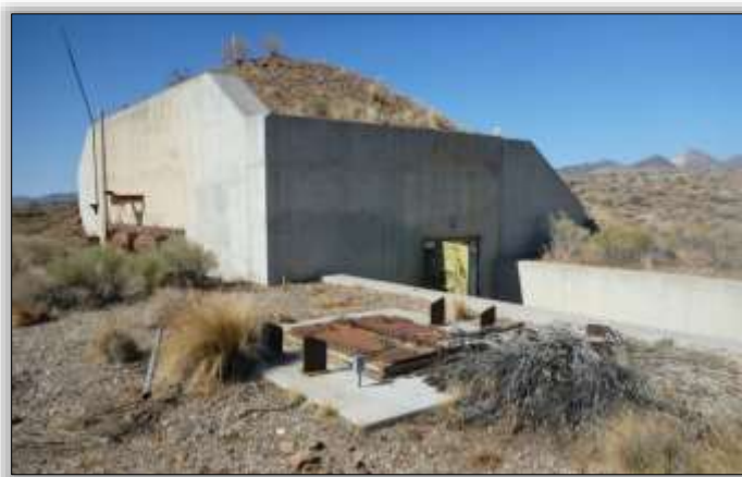
Fast Photo Bunker used during the Shasta test in 1957. The Bunker was designed to record reaction speed of nuclear detonations and held an electronic streak camera cable of recording images in one billionth of a second.
