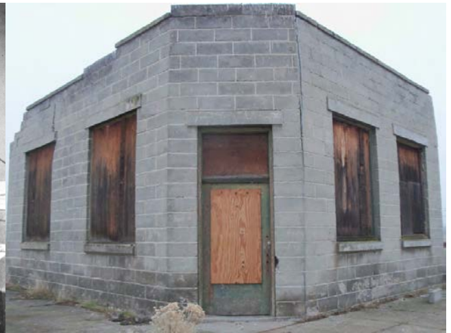
Main entry at the northwest corner; September 2012.
