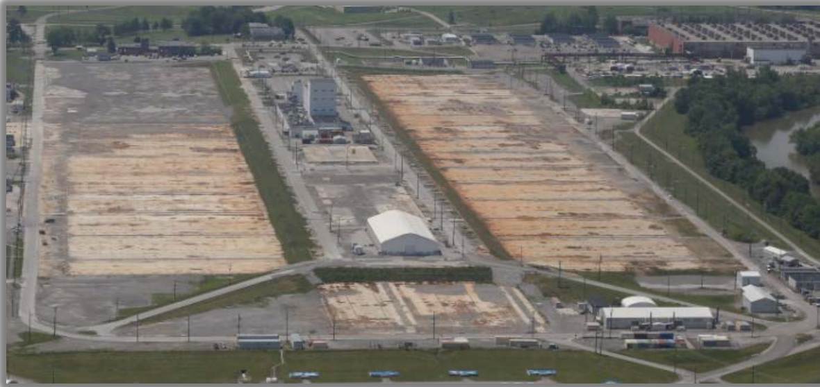
K-25 Building Slab
