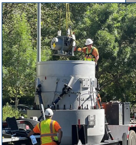
Removal of a cesium irradiator through CIRP.
