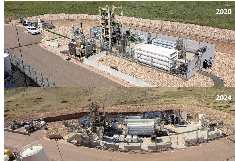
NREL HITRF Station Expansion from 2020 to 2024
